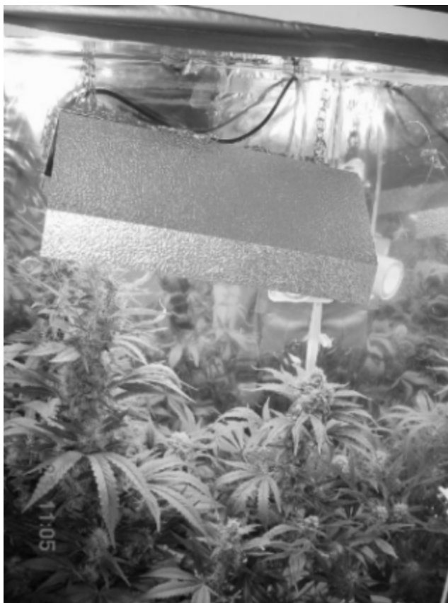
Figure 3.4 - This is a great picture of an indoor grow room by GIYO. The light hanging down over the plants is a HPS light. It gives off an orange glow to the grow room.
