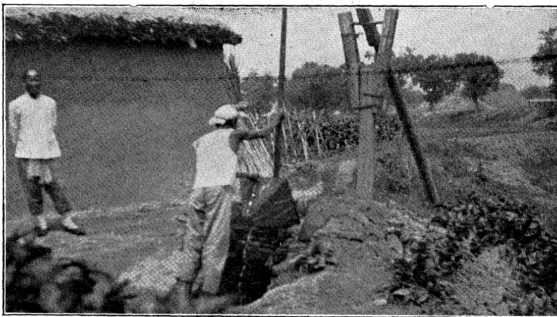
Fig. 170.—Well sweep and quadrangular, conical water bucket used for irrigation in Chihli.
