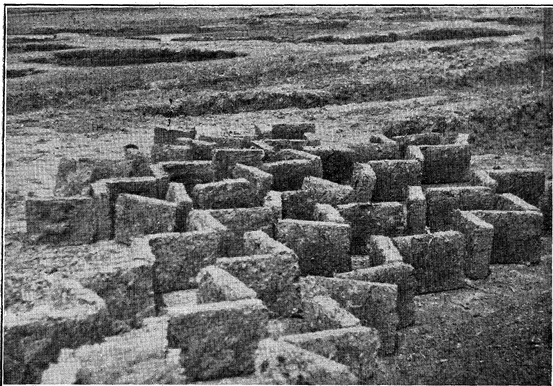
Fig. 89.—Air-dried earth brick for house building.
