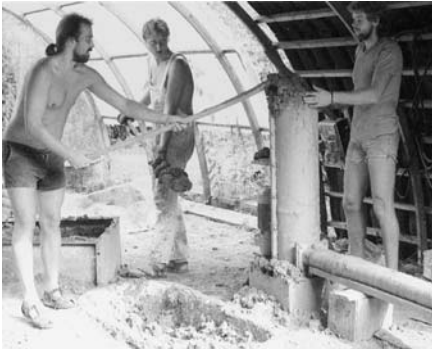
Preparing the mix
