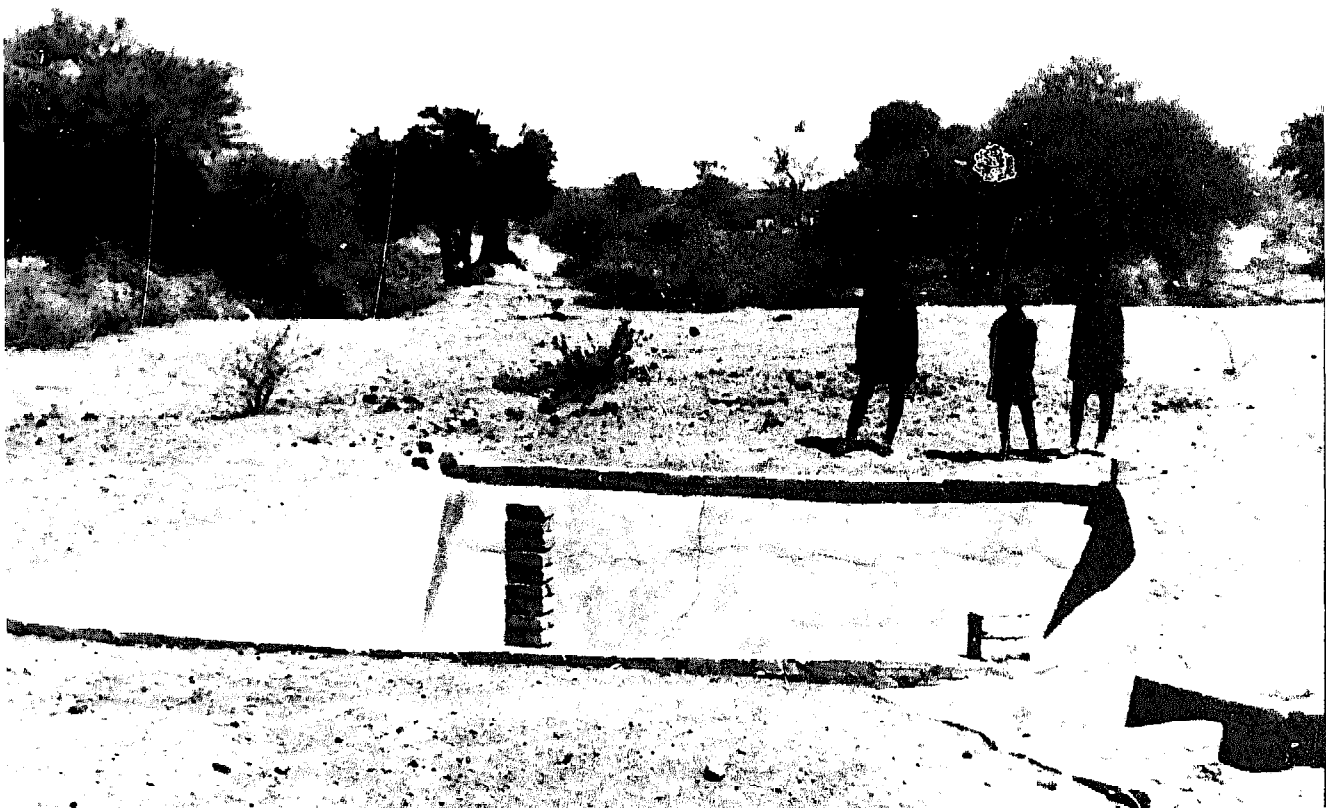
Plate 6. An excavated brick-and-cement ground catchment tank of 50 cubic metres at Morwa, near Gabarone, Botswana. (The tank was financed by money raised by the children through the school fund and the free labour of a local builder.) The tank waters the school garden in the dry season. (John Gould)
