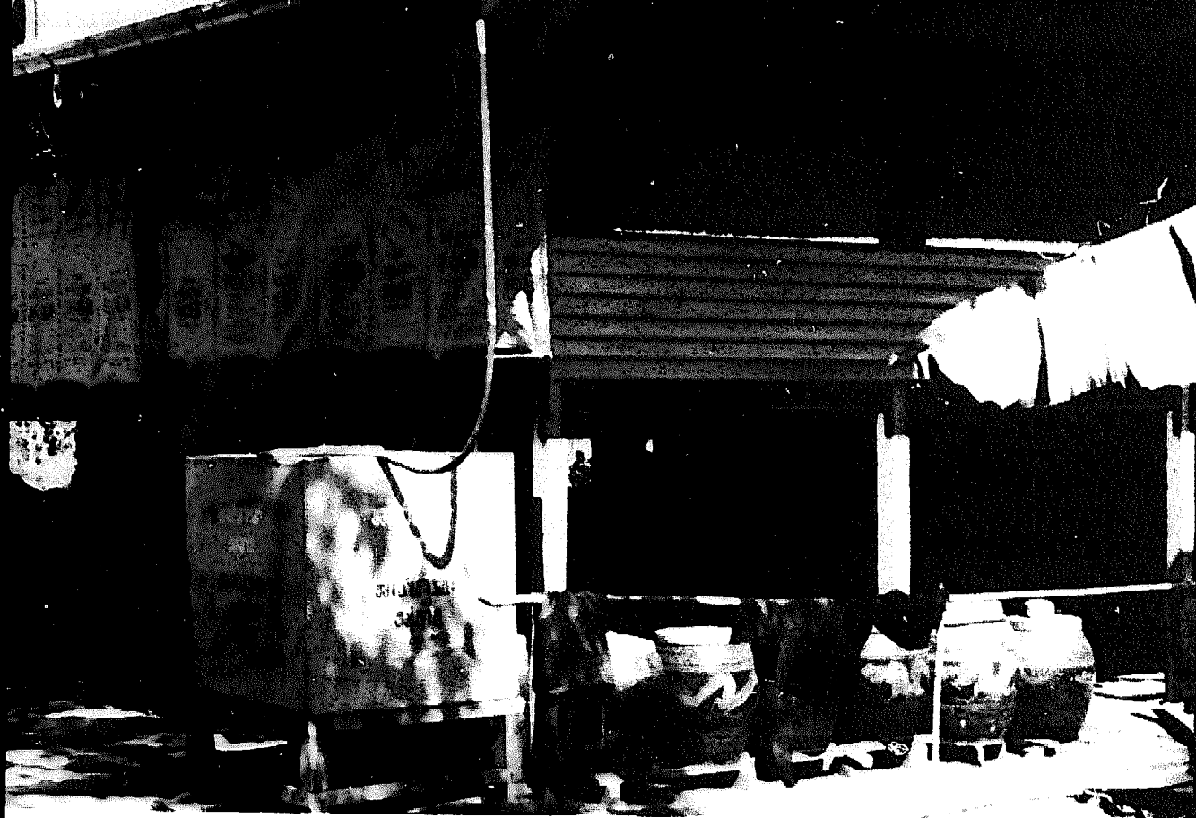
Plate 1. The methodical collection of rainwater in the domestic system of a fairly affluent family in Thailand, showing funnel/filter and a flexible pipe filling the galvanized tank. (Alongside can be seen the traditional decorated clay jars, called 'dragons' fitted with lids.) (John Collett)
