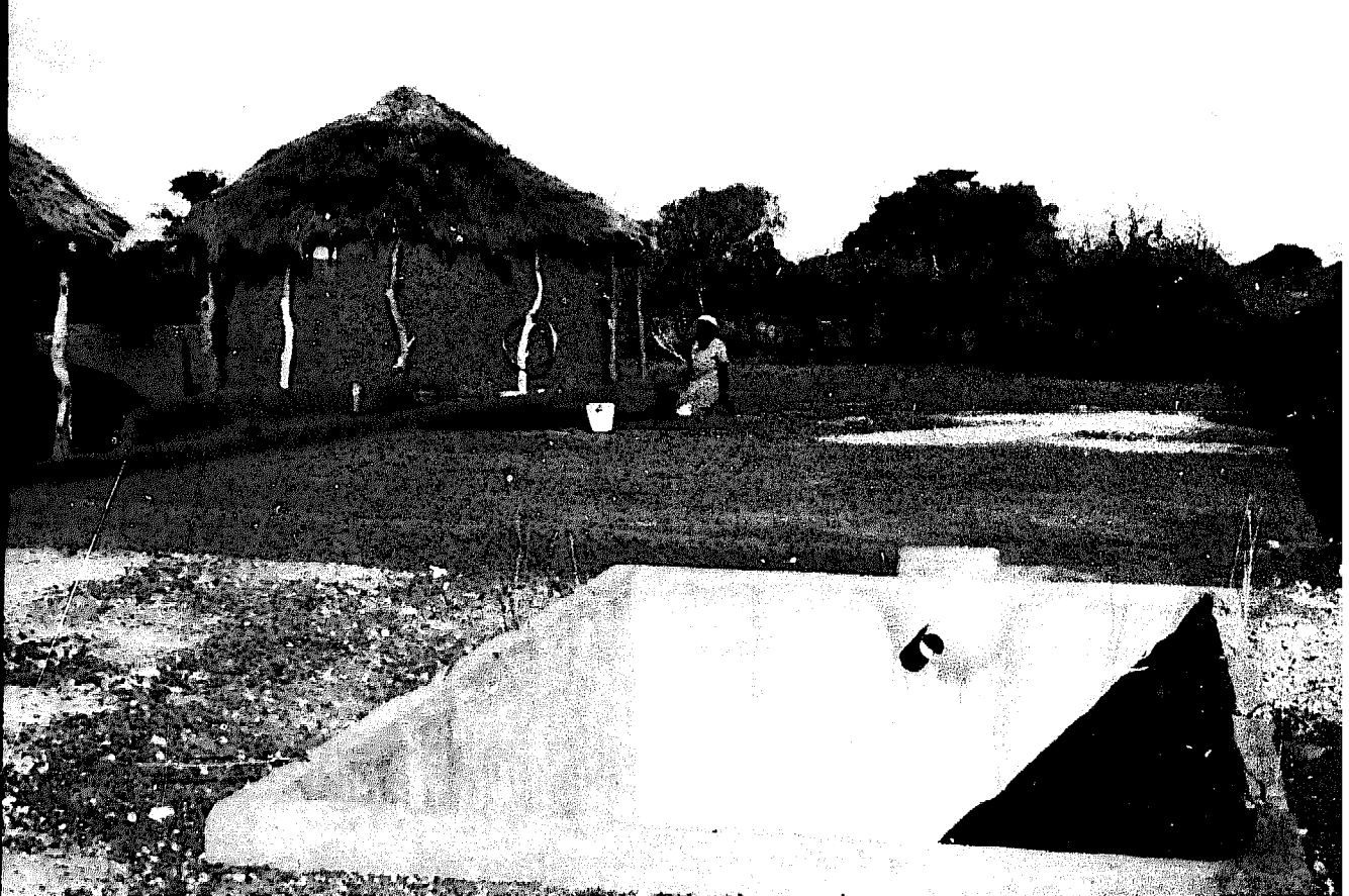
Plate 8. A brick and cement rainwater catchment tank at Pelotshetla. In the background a woman can be seen smearing the threshing floor catchment apron with a mixture of dung, water and mud. (John Gould)
