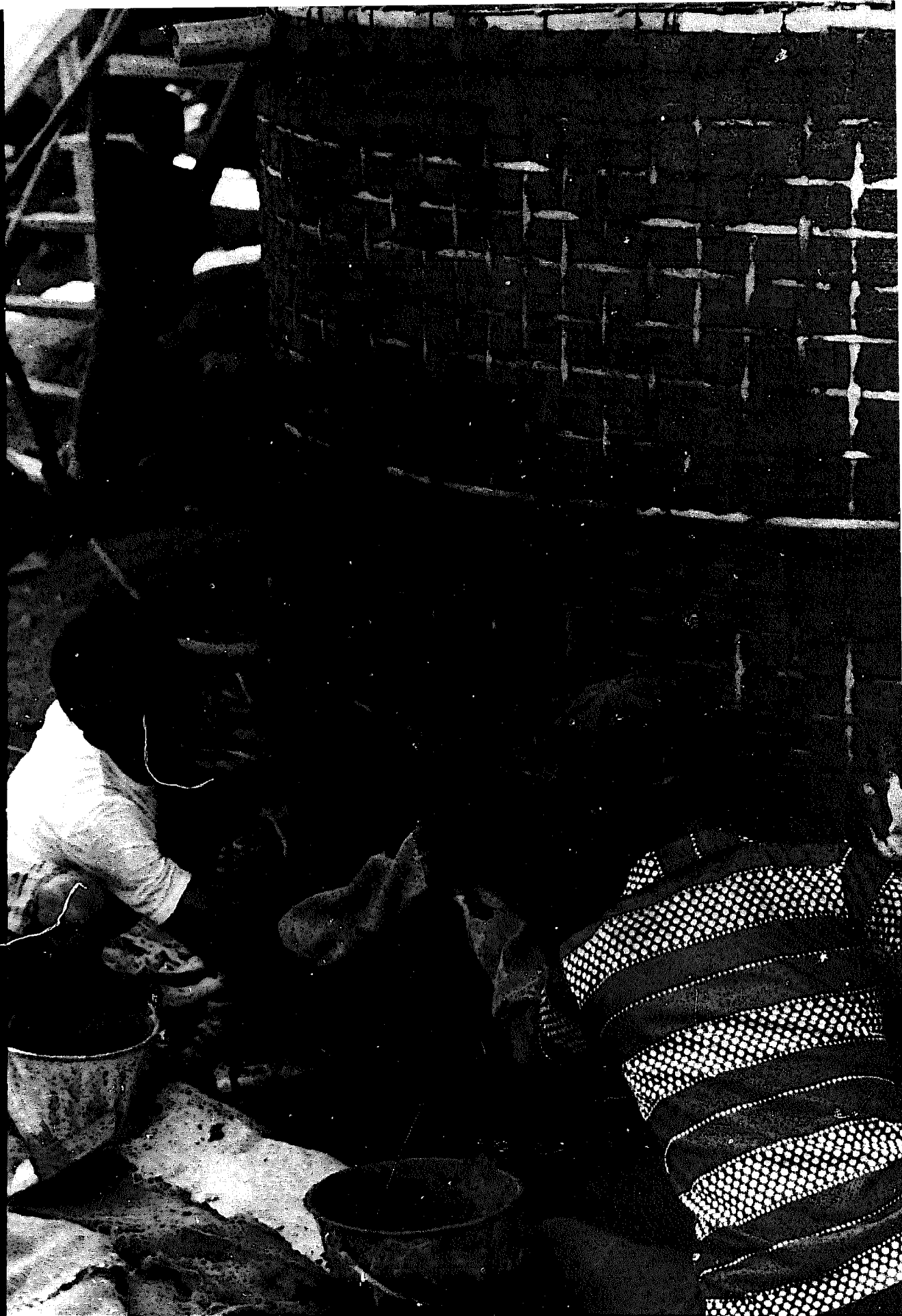
Plate 9. A bamboo-cement water tank, Indonesia, being plastered. The walls and floor of the tank are plastered first inside, then outside. (Ben Young)
