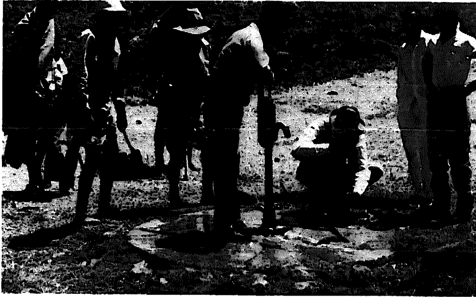
Student sanitarians check and repair a well near the Kolladuba Health Centre in Ethiopia. (photo: WHO)
