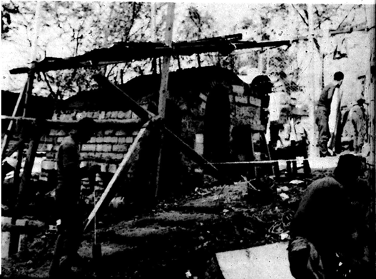
199. View during construction.
