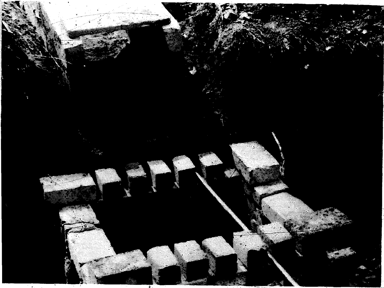
178. Construction of the firebox and ware chamber. The notches will hold the metal grate rods.
