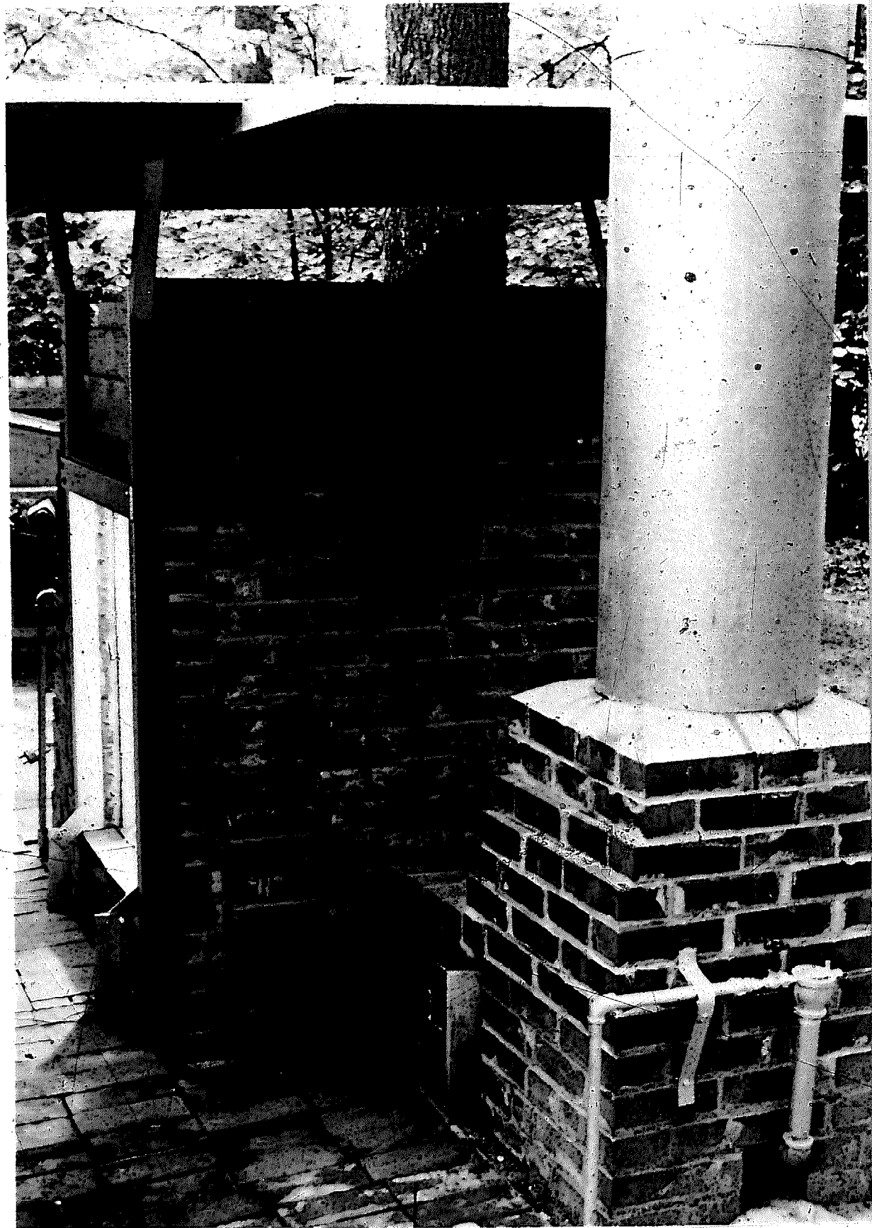
127. Stack. A burner is provided to warm the stack and induce a good draft for the early stages of firing.
