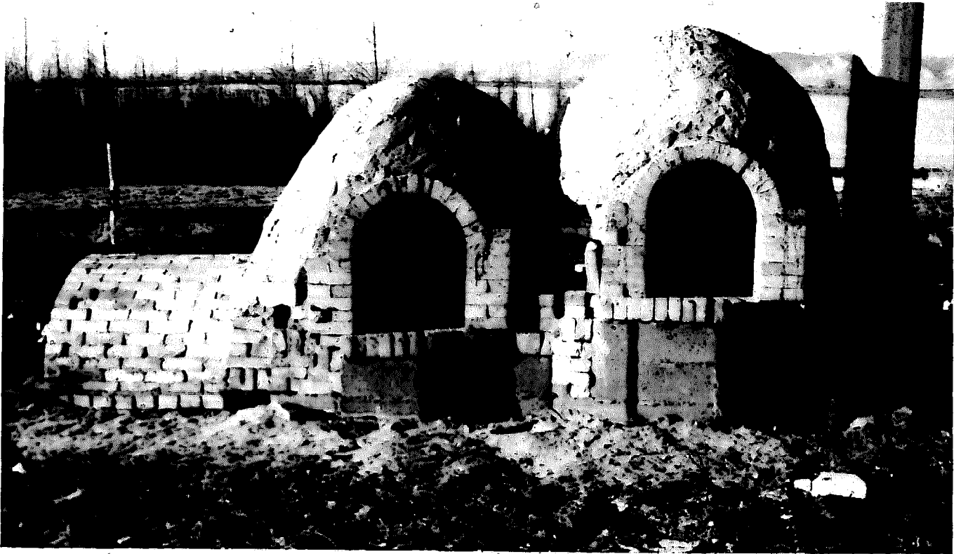
61. Two-chamber wood burning kiln built by William Alexander at Ft. Collins, Colo. The domes were made of cone-shaped brick made especially for this kiln.
