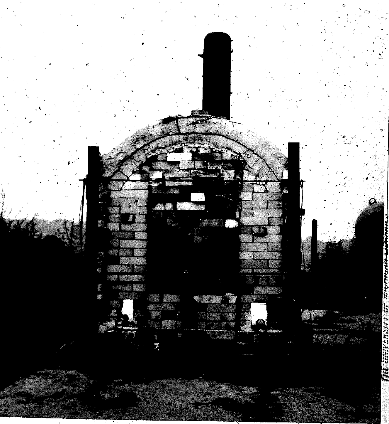
93. Don Reitz kiln firing on liquified petroleum gas. A second layer of brick has been added to the side walls and arch.
