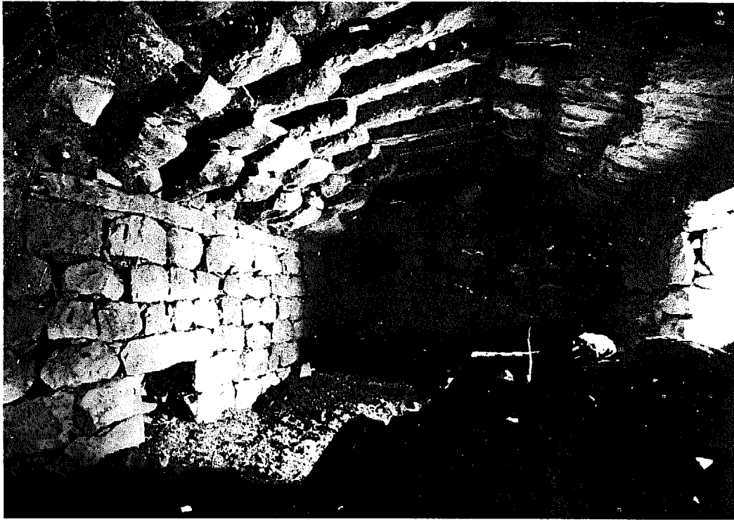
Above: Basalt stones, quarried locally, were used to build this interesting corbelled roof from Syria. Below: The Inca base of a building in Cuzco, Peru, achieves remarkable fit without the use of cement or mortar.
