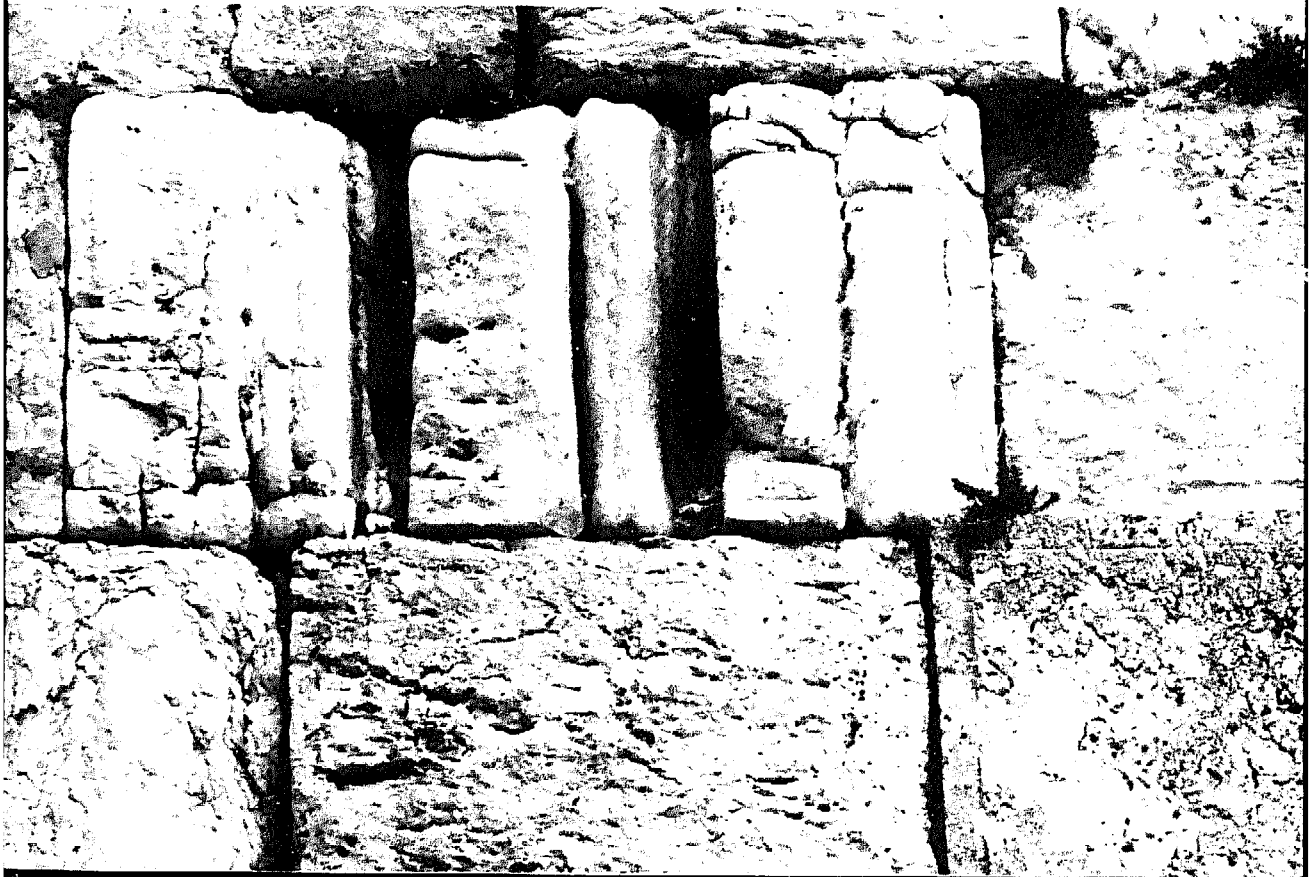
The use of slate need not be confined to roofs! Above: Laying a slate damp-proof course, Nepal. Below: Stone that was edge-bedded during construction has suffered from weathering, while the naturally bedded stone surrounding it is in far better condition.
