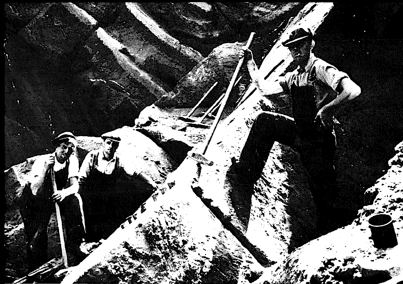
Above: Splitting sandstone by wedge in Scotland
