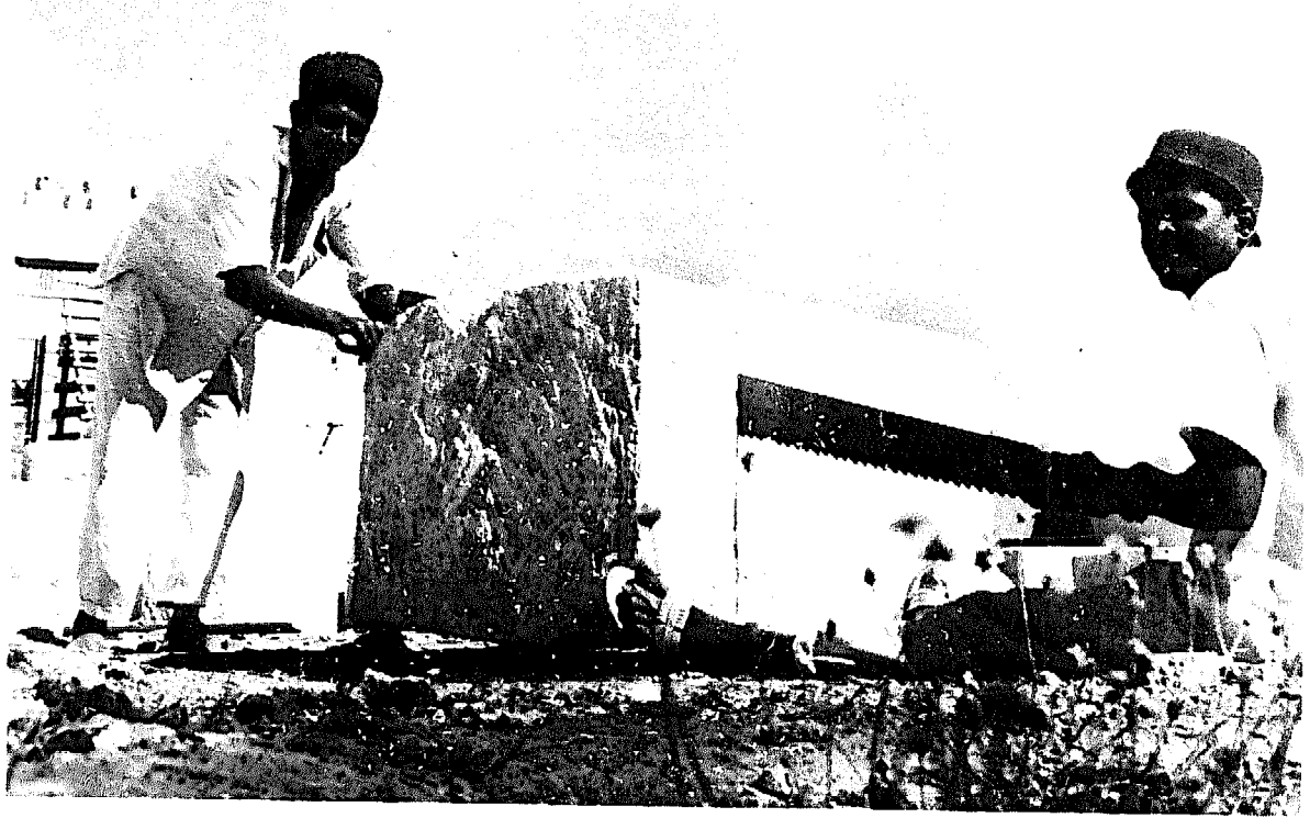
Above: Sawing limestone into building blocks; but industrial blocks have to conform to exact measurements.
