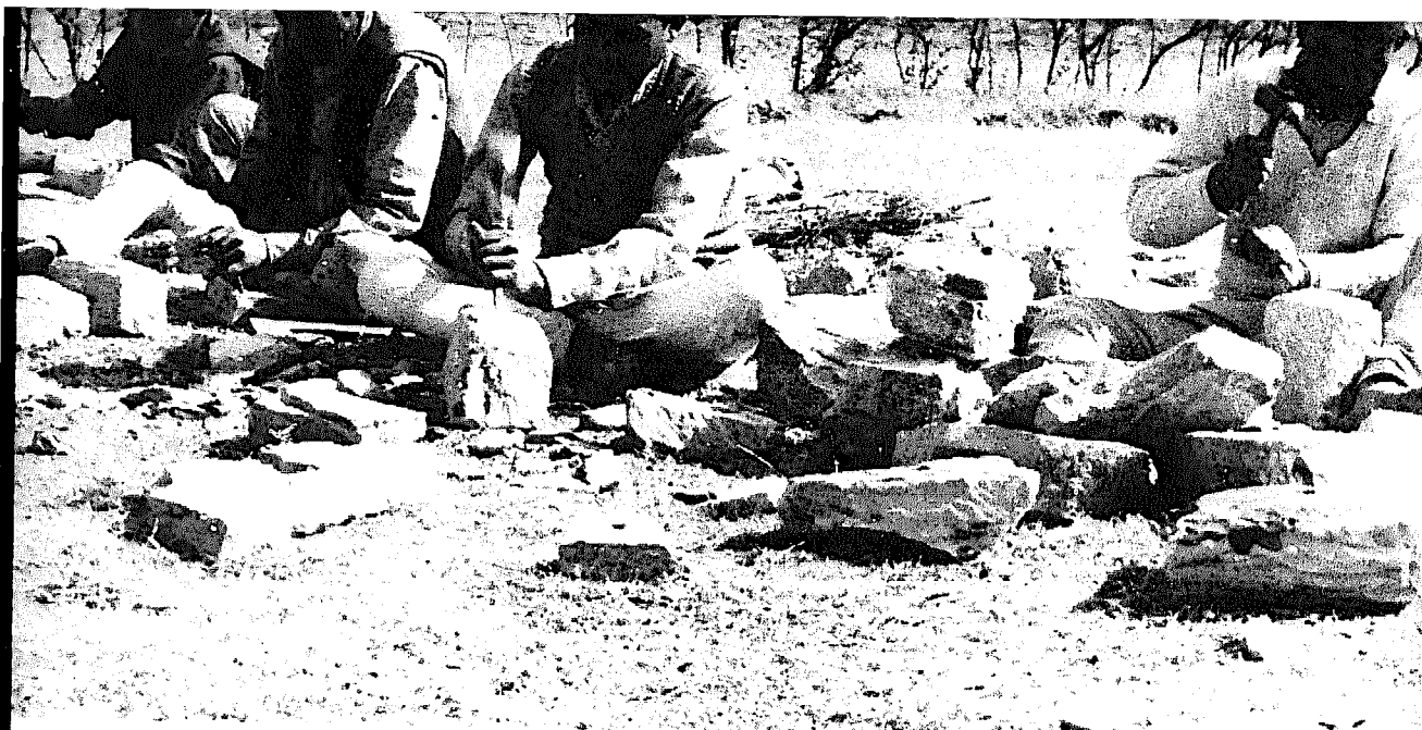
One of the greatest advantages of stone is that it can be shaped using a hammer and chisel (above). Once squared, blocks can be used to build simple buildings, such as this dry-wall dwelling, from Argentina (below).
