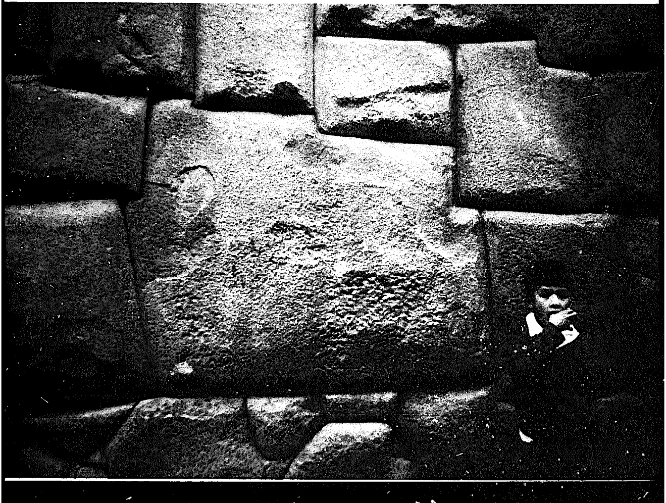
Above: Basalt stones, quarried locally, were used to build this interesting corbelled roof from Syria. Below: The Inca base of a building in Cuzco, Peru, achieves remarkable fit without the use of cement or mortar.
