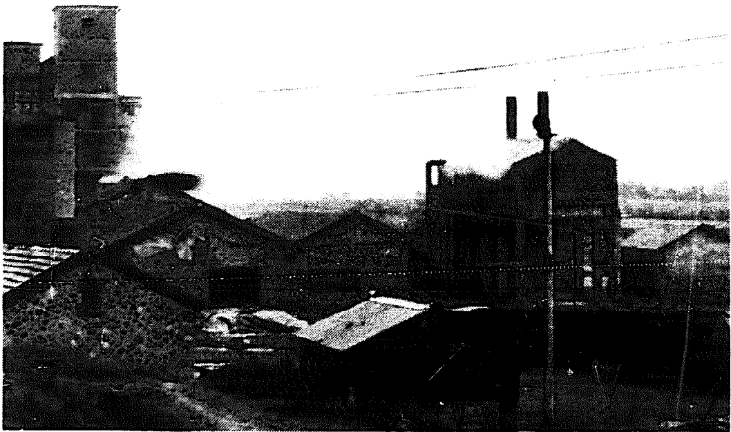
Fig 2. Small scale cement plant, China Capacity 100 tonnes/day
