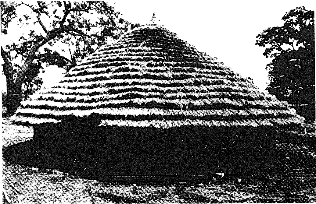
Completed "case" (traditional round house)
