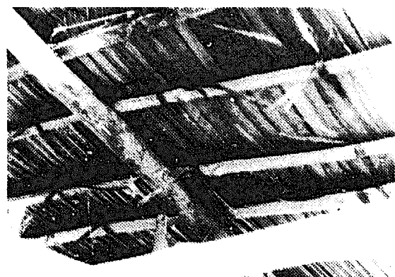
Production and installation of Raphia palm leaf tiles, Ghana (Photos: H. Schreckenbach, Bibl. 00.49)
