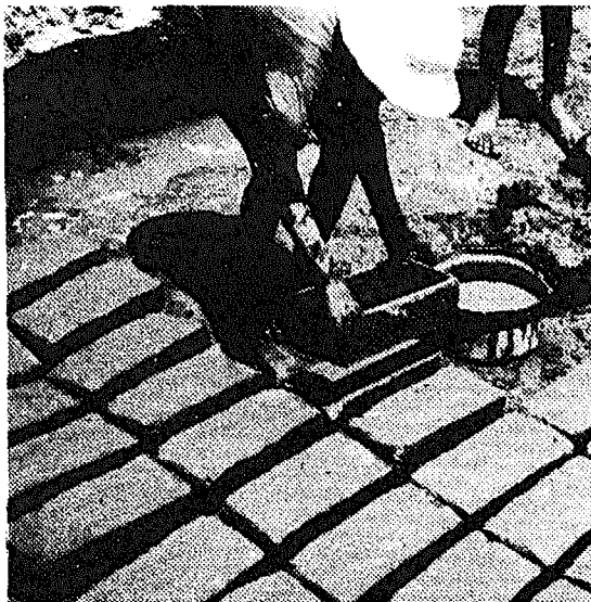
After smoothing the top surface, removal of the mould
