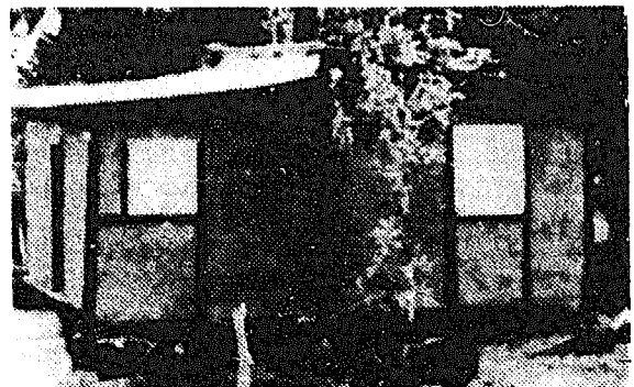
Completed ferrocement house
