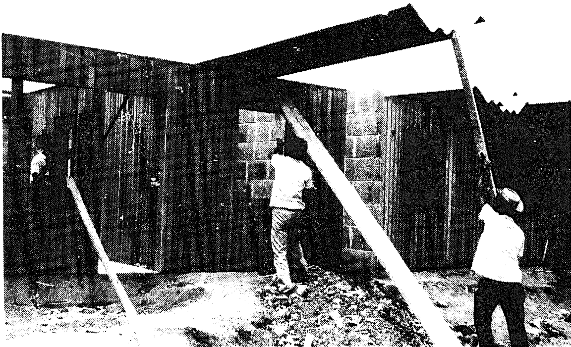
Placing a Canaleta roof in Tegucigalpa, Honduras, 1967: rapid installation by unskilled labour (Photo: Alvaro Ortega, who developed this roofing system).
