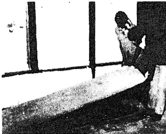
Lifting of the finished roofing element from the mould; assembly of two elements
