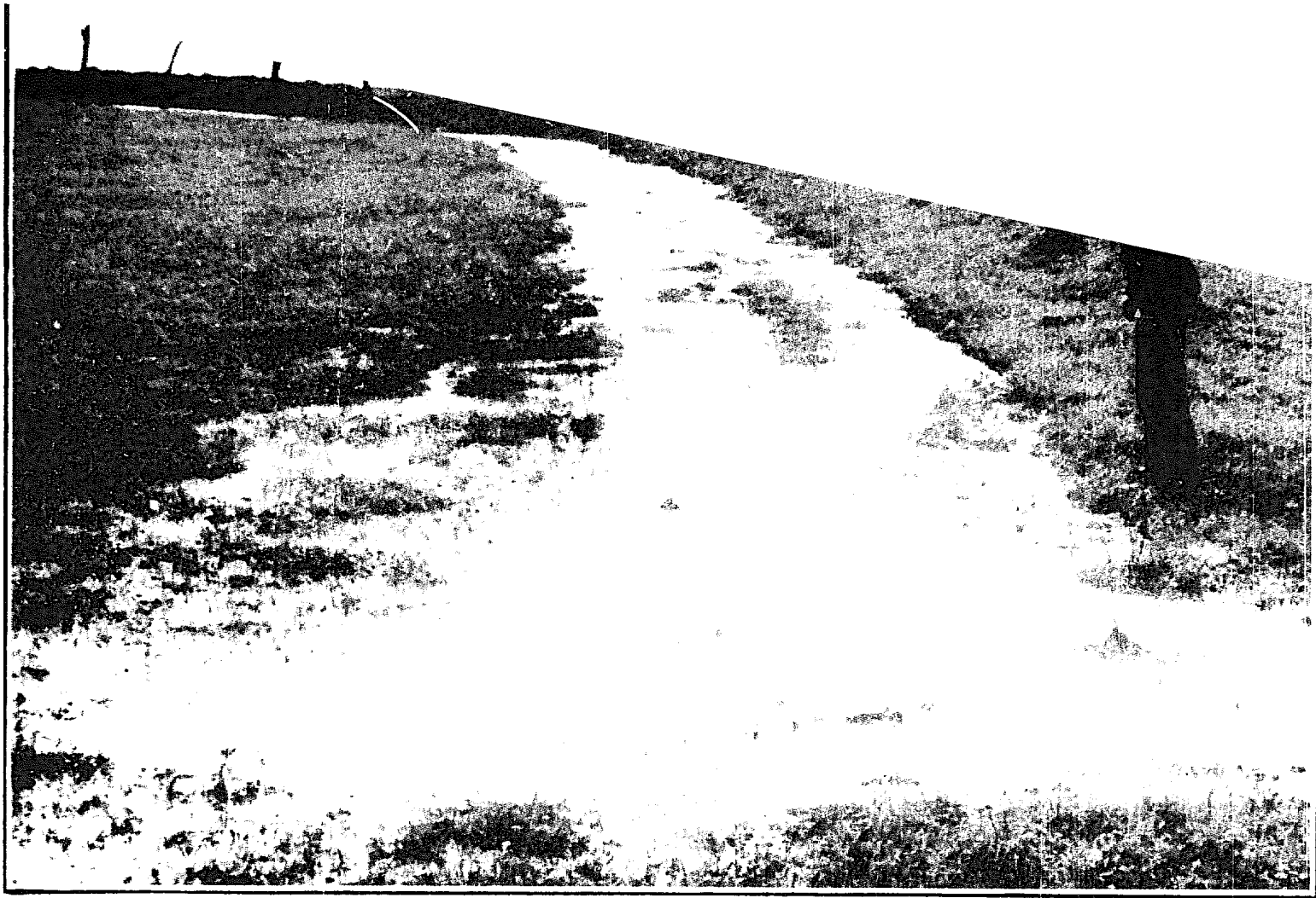
FIG. 132. An inch of rain fell in Haskill Co., Oklahoma, in half an hour. A terrace pours its surplus into a grassed channel that will not erode, and spreads the water over a pasture. (Photo Hufnagle, U. S. Soil Conservation Service.)
