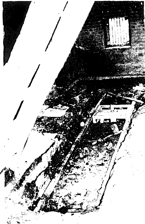
First stage of installation of another MPPU set-up.
