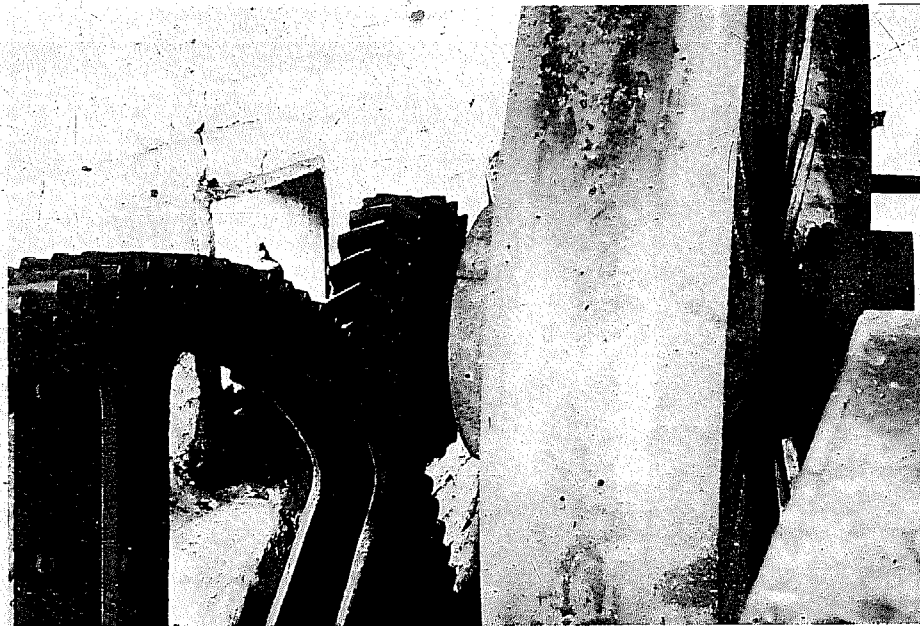
Fig 2.57 Close-up of the first stage of gearing for the sawmill in fig 2.53, showing double helical gearing, which is unusual for a watermill but is probably a relic of the former use of this mill for paper making
