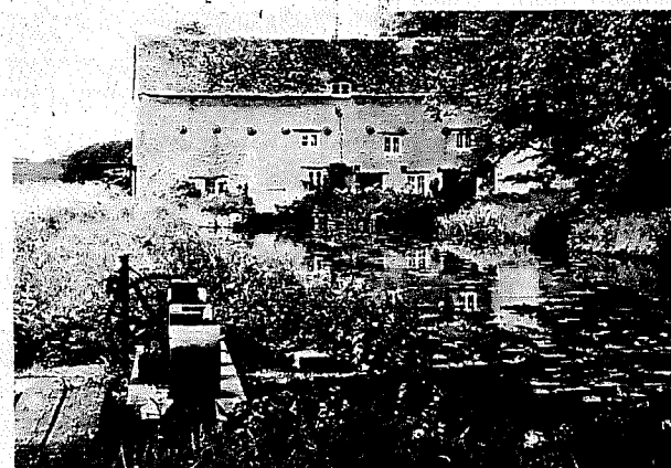
Fig 1.27 Wadenhoe Mill, near Oundle, Northamptonshire. The mill is situated on an artificial cut or leat and the main stream of the River Nene is navigable at this point. In the right foreground is the sluice for diverting water into the by-pass channel
