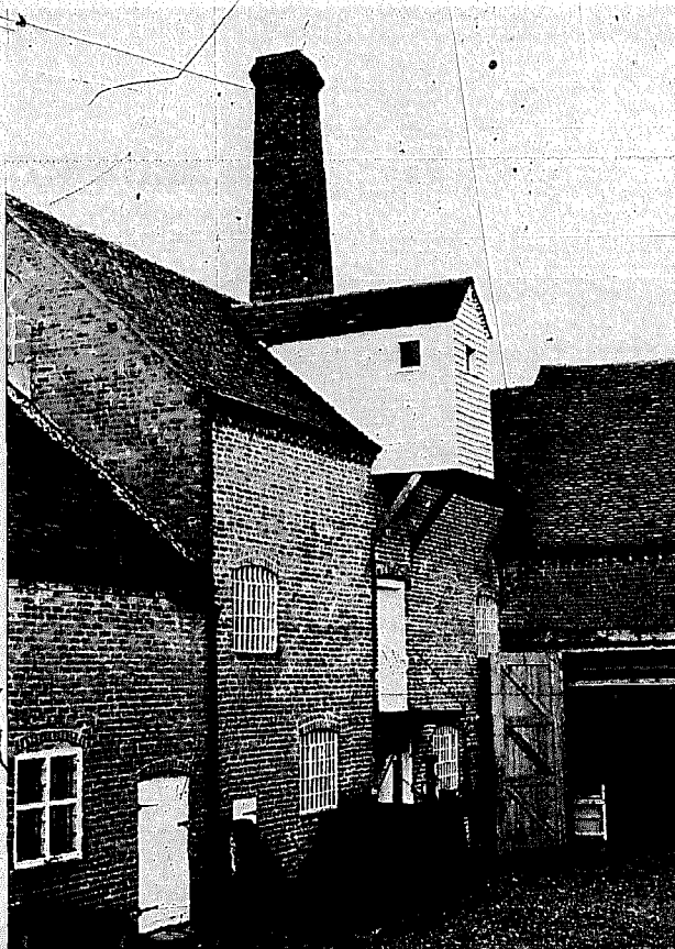
Fig 1.81 The white weather-boarded lucam, covering the external hoist, protruding from the roof at Sarehole Mill, Birmingham
