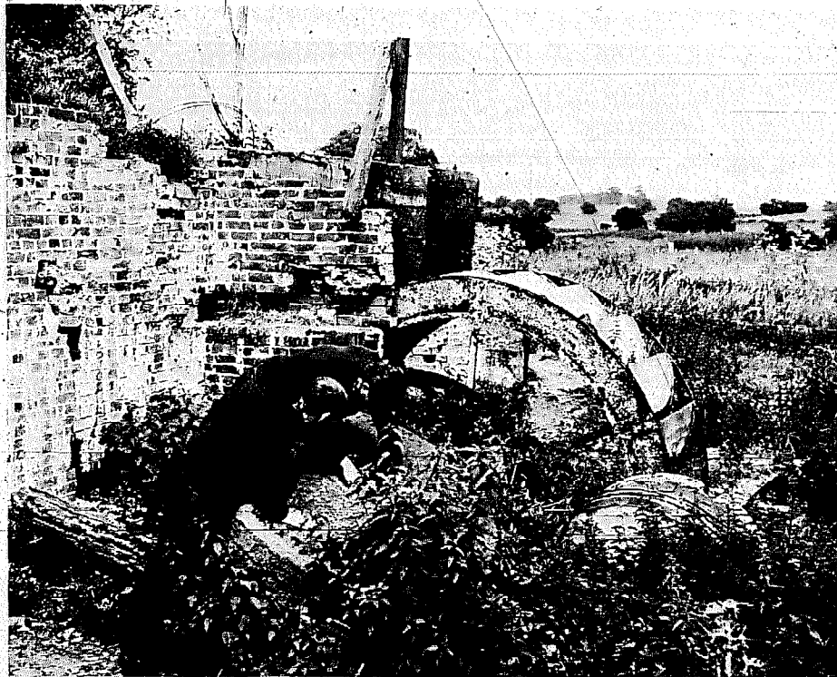
Fig 1.33 Overshot waterswheel in the ruined mill close to Churchover, near Rugby, Warwickshire. Note the remains of the wooden launder and 'shut' for bringing water onto the top of the wheel
