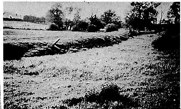
Fig 2.9 The artificial leat, made to serve Maidford Mill, on a tributary of the River Tove in Northamptonshire. The pentrough onto the overshot waterwheel is off the left of the picture. The natural course of the Maidford Brook is shown by the line of low hedges just in front of the field with sheep in the left background
