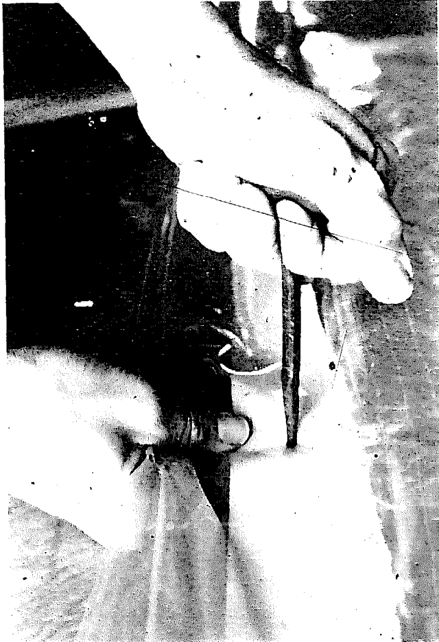
Photo 8-23: Batt covered with polyethylene.
