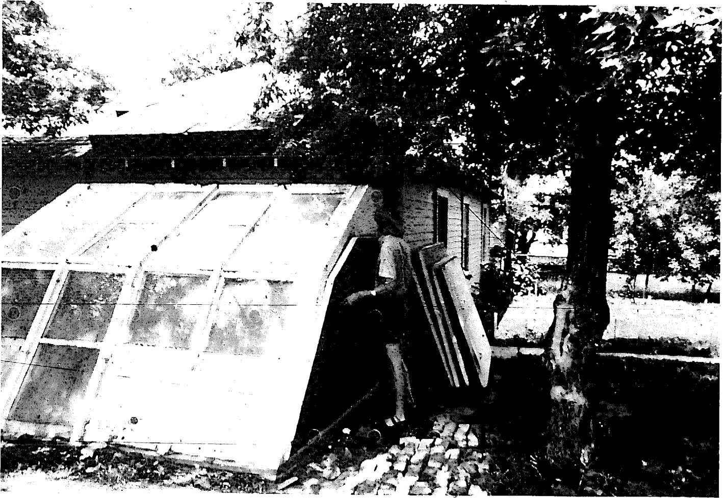
Photo 9-9: Solar greenhouse attached to garage. Note solar collector on roof. Milwaukee, Wisconsin.
