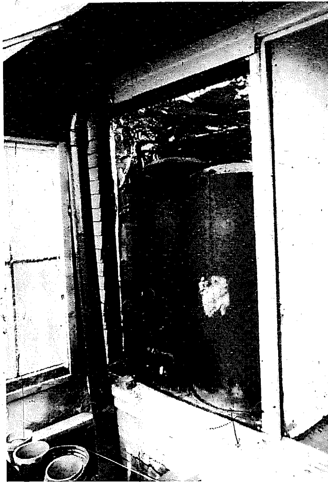
Photo 5-7: Water storage. Used water heater. Milwaukee, Wisconsin.
