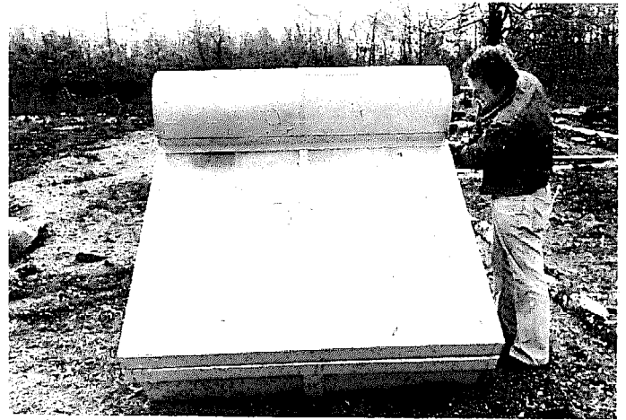
Photo 11-5: Insulation filling glazing.
