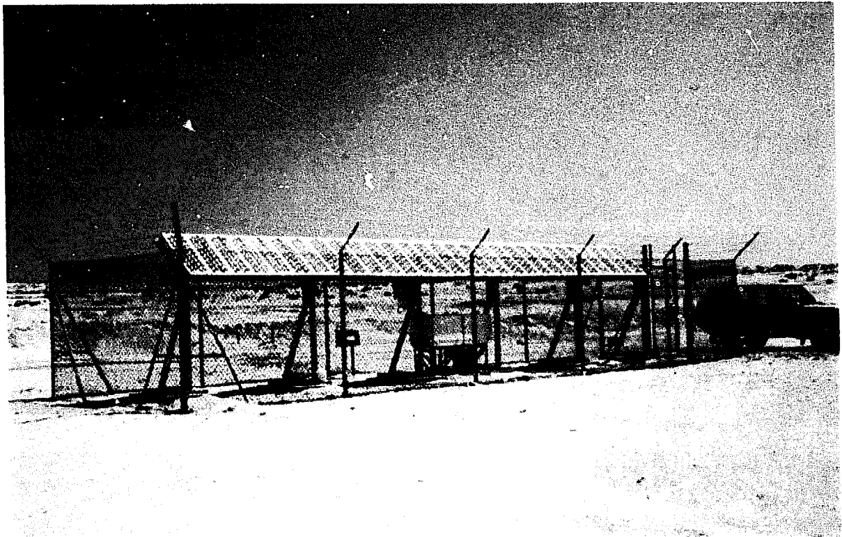
Figure 7.2 PV-powered Cathodic Protection System for Pipeline in Abu Dhabi
