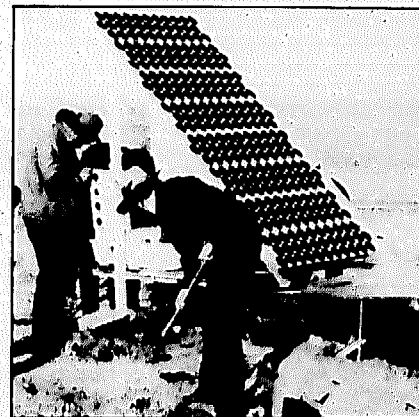
Workers put the finishing touches on a unique PV installation in Utah which controls highway warning signals. To bring in the power lines would have cost the state 125,000 dollars.
