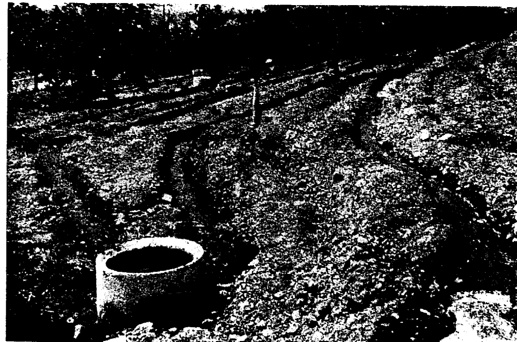
Fig. 24. Irrigation Water supplied to furrows by hydrants using slide gate outlets
