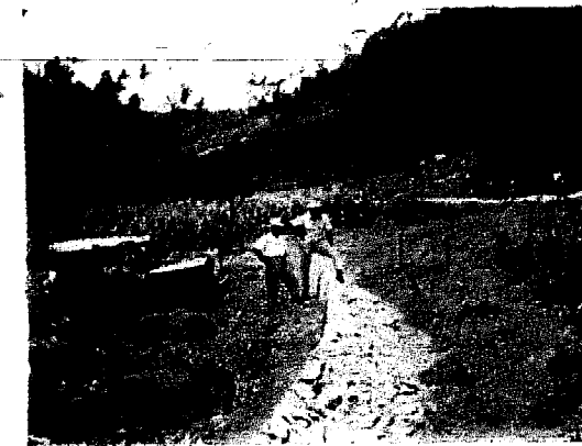
15. Erecting stone barriers. Slope them back into the hill
