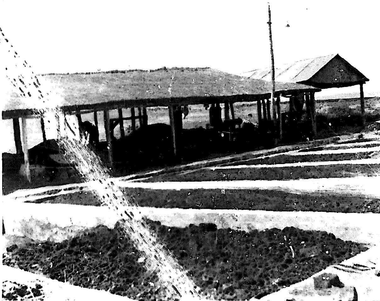
FIG. 27. MUNICIPAL COMPOST PITS WITH COVERED HAMMER-MILL AND SCREENS AT FICKSBURG, ORANGE FREE STATE
