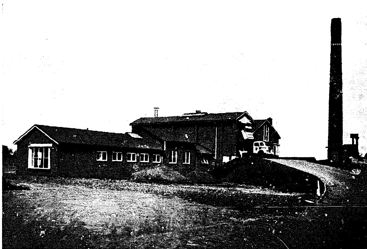
FIG. 26. COMPOST PLANT AT SCHIEDAM, NETHERLANDS
