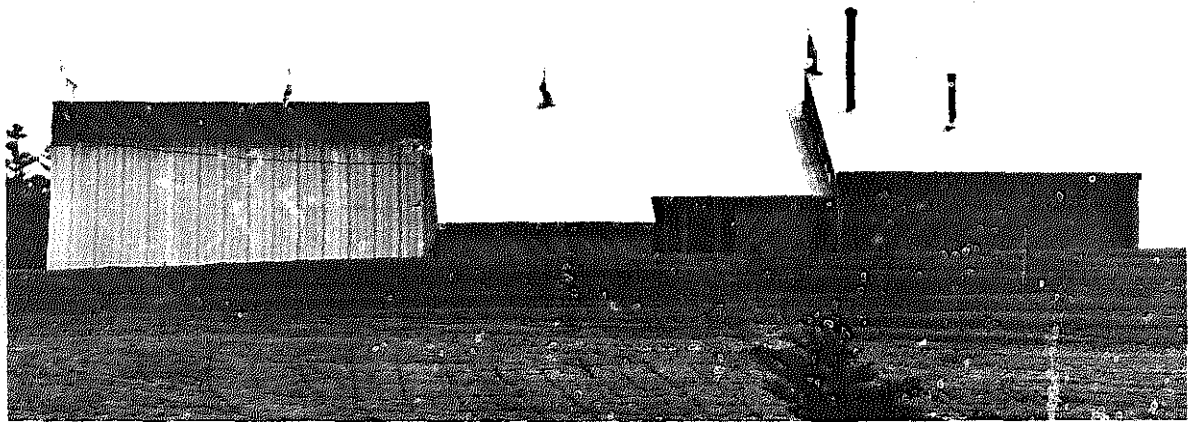
Photo 2 -- North Side of the Ark, with Berm in Foreground
