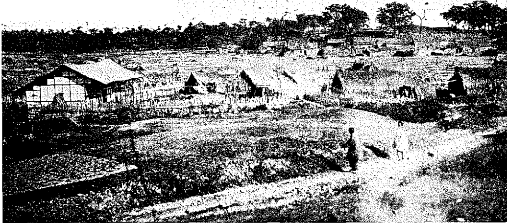
FIG. 1. A CHINESE COAL MINE. Surface structures of a coal mine at Kong Tong, Kiangsi. Thatched straw huts, the miners' dwellings, are built over the mine shafts. A large half-timbered house is seen to the left.
