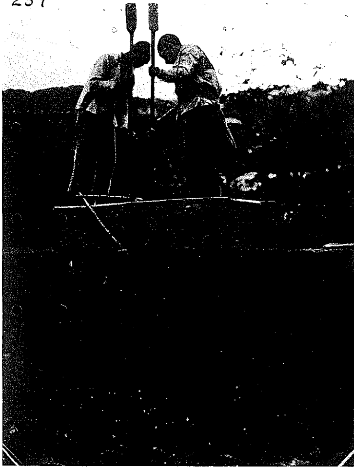
FIG. 439. TWO MEN RAMMING EARTH INTO A SHIFTABLE WOODEN FORM, IN BUILDING A WALL OF PISÉ DE TERRE.
