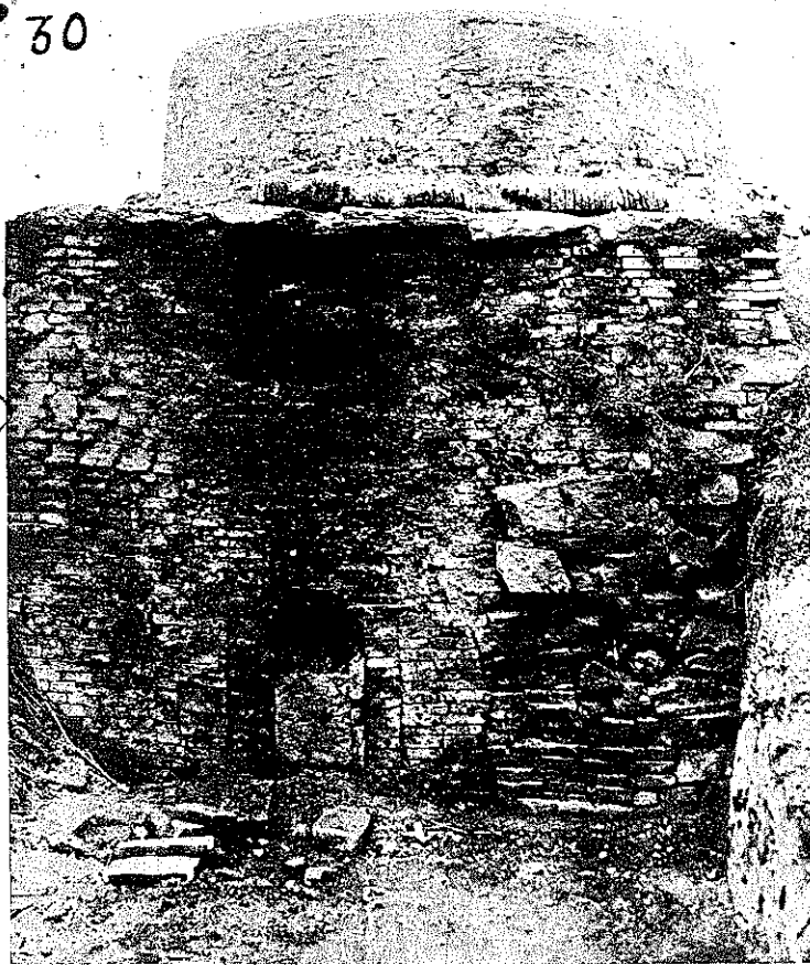
FIG. 388. BRICK KILN SHOWING FIRING HOLE.
