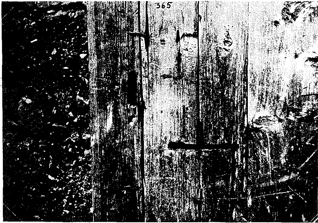
FIG. 452. DOOR LOCK, OUTER SIDE. The vertical, upper slot is for insertion of the key and releasing the bolt from its tumblers, and the lower horizontal slot for the push pin to prick and slide the wooden bolt sideways to open the door. Key and push pin are shown in Fig. 453.
