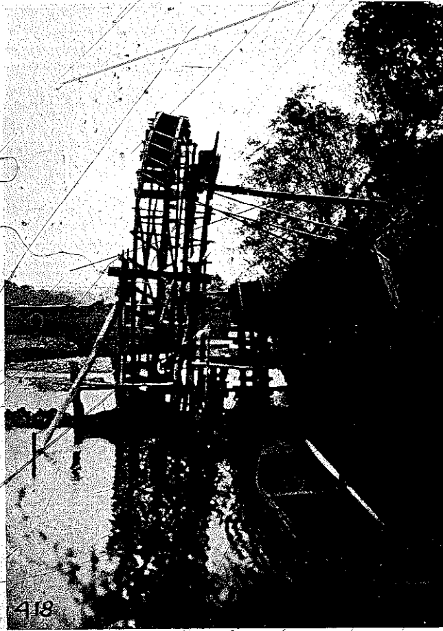
FIG. 175. UNDERSHOT WATER-WHEEL FOR RAISING WATER.
