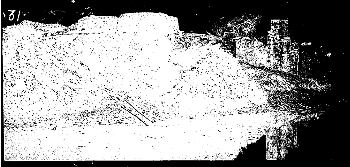
FIG. 389. FUEL OF PINE BOUGHS, USED FOR BURNING BRICKS, AT BRICK KILNS SEEN IN BACKGROUND.
