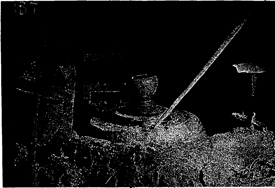
FIG. 520. POTTER'S WHEEL FOR MAKING SMALLER EARTHENWARE.
