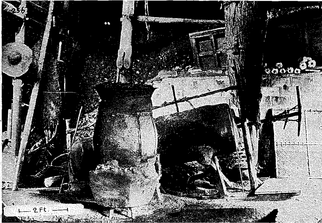
FIG. 41. IRON CASTER'S FURNACE.
