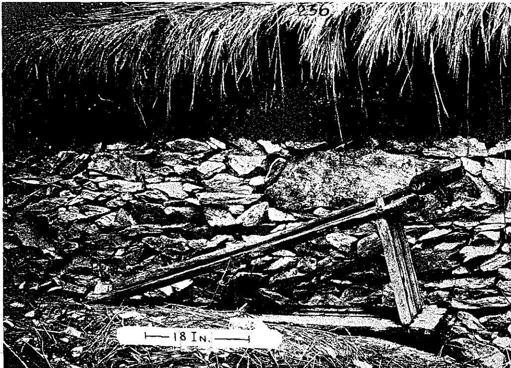
FIG. 438. WOODEN FORM AND RAMMING STICK USED TO BUILD A PISE DE TERRE WALL, HERE SEEN PARTLY BUILT, RESTING ON ITS STONE FOUNDATION.
