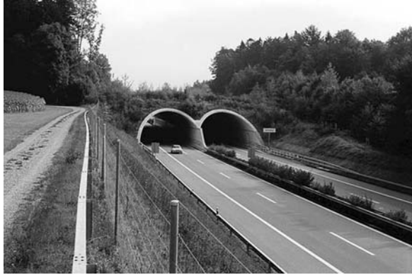
Fig. 5.2 Overpasses allow some animals to move freely between habitat patches and avoid the hazards of crossing busy highways. Photograph by Scott Jackson
