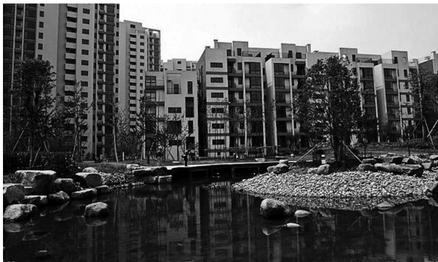
Fig. 15.3 Skyscrapers. An example of an ecologically designed residential compound. From now on, almost all Jiaxin's newly built residential areas are designed and planned with ecological and energy-saving considerations
