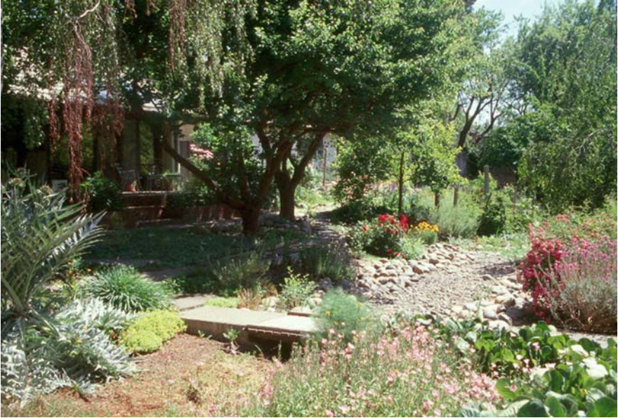
Fig. 4.2 Natural drainage system at Village Homes in Davis, CA
