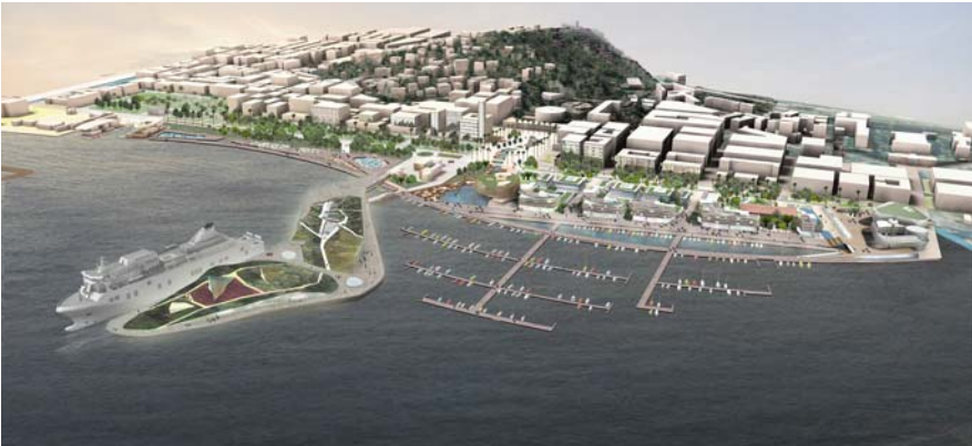
La Spezia, Italy © Arup
