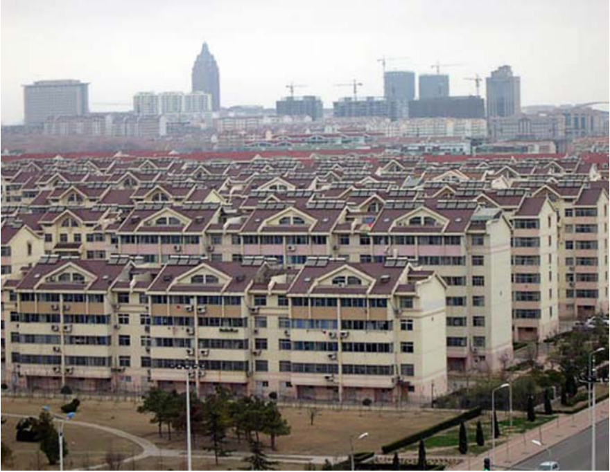
Fig. 14.3 Rizhao rooftops with solar thermal water heaters [11]
