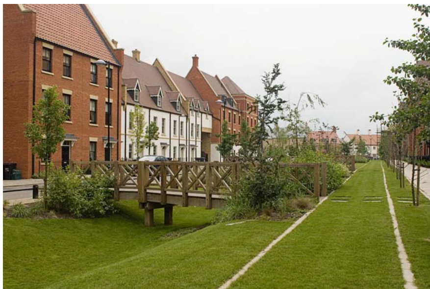
Fig. 10.3 Upton's sustainable urban drainage system is integrated with its public spaces
