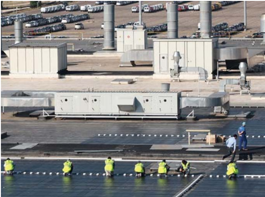
Solar array being installed on a General Motors assembly plant in Zaragoza, Spain
