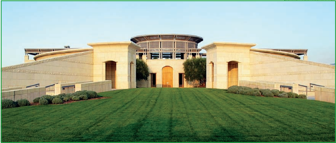
The Opus One Winery in California's Napa Valley was not conceived as a green building in the early 1990s. However, the building captures many elements of today's green designs: partially underground for insulation and cooling, use of daylighting, natural materials, and water conservation. (Chuck Szmurlo)
