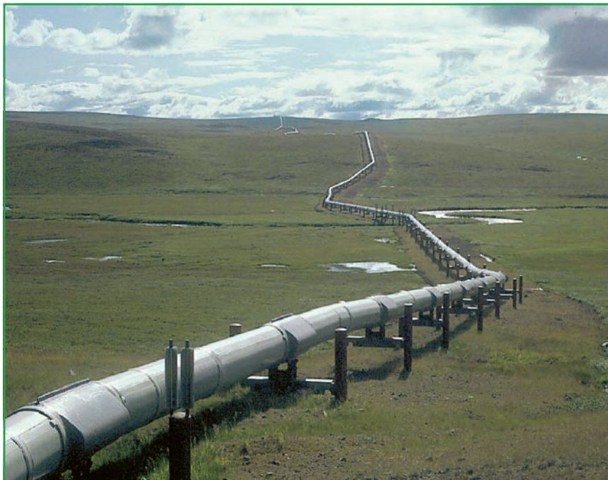
The Trans-Alaska Pipeline at Kuparuk on the Alaskan Arctic plain. In 2006, the pipeline ruptured and spilled more than 270,000 gallons (1 million l) of oil into Prudhoe Bay. Cleanup teams struggled in temperatures of -63^{\circ}\text{F} ( -52.8^{\circ}\text{C} ) to dislodge oil frozen to ice. The spill rekindled debate over proposed drilling in Alaska's Arctic National Wildlife Refuge (ANWR). (William Breck Bowden)
