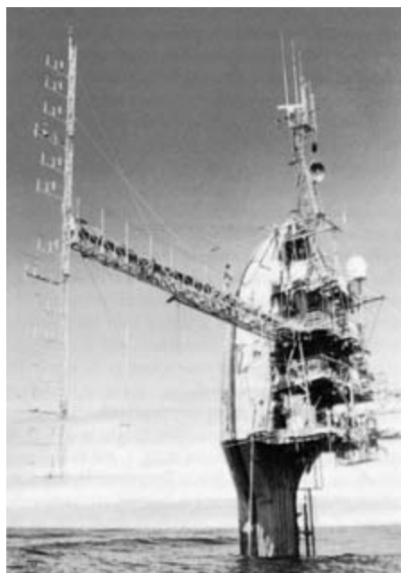
Fig. 6.13 The stable FLIP platform for measurement of wind velocity/boundary layer data in the offshore environment 50 km west of Monterey, California.
