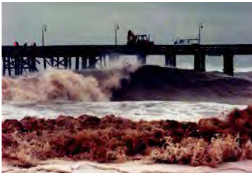
Heavy rains in Southern California damaged the Ventura Pier during El Niño–driven storms in 1997 and 1998. AP IMAGES.
