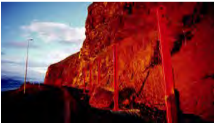
Beams and wire netting form a rock slide fence near Bolungarvik, Iceland. ©PAT-RICK BENNETT/CORBIS.
