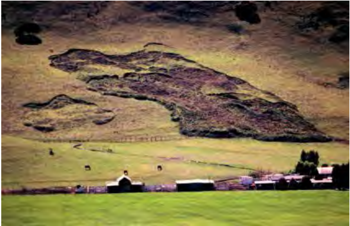
A landslide approaching farm buildings in California. JLM VISUALS.
