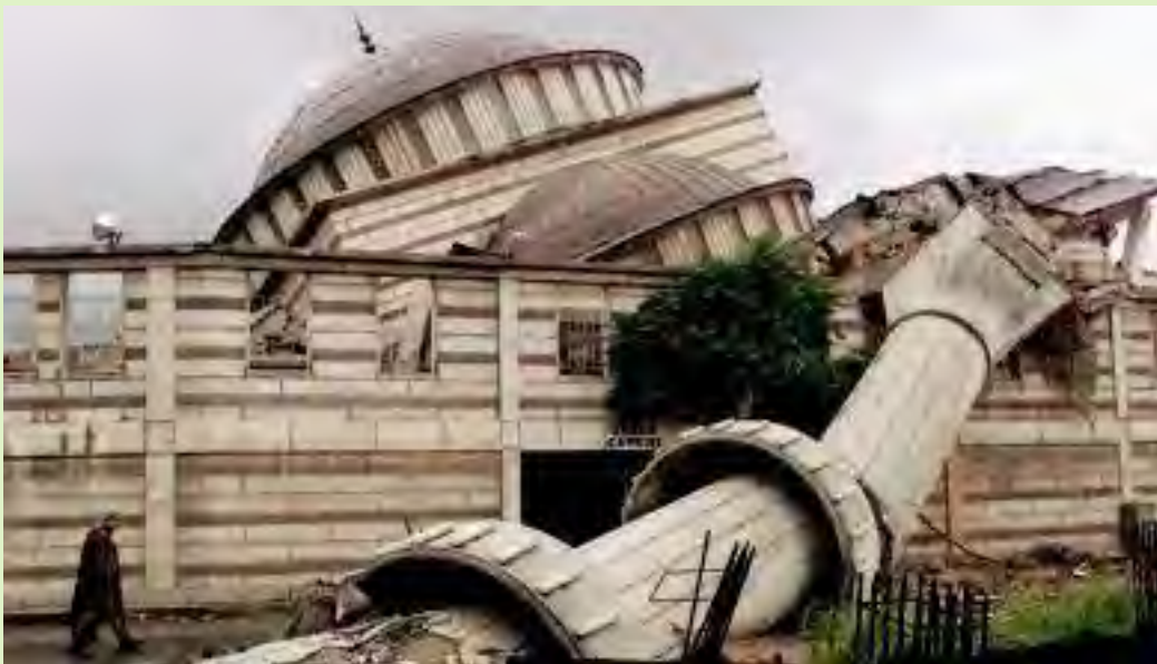
Earthquake damage to a Turkish mosque, 1999. ©SERGEI CHIRIKOV/EPA/CORBIS.
