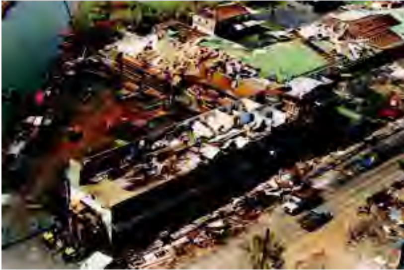
Buildings in downtown Kapaa, Hawaii, rest with their roofs split open in the aftermath of Hurricane Iniki. ©REUTERS/CORBIS.
