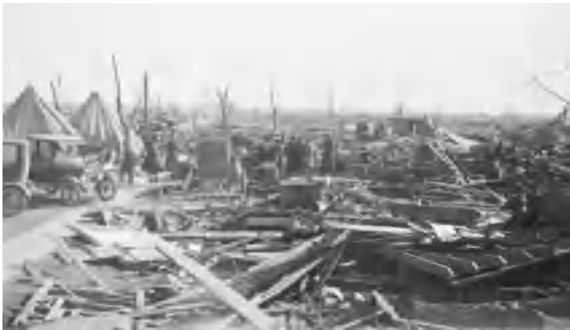
Men survey damage done by a tornado that moved through Griffin, Indiana, in 1925. ©BETTMANN/CORBIS.
