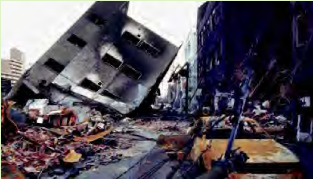
A section of Kobe, Japan, demolished by the 1995 earthquake. ©MICHAEL S. YAMASHITA/CORBIS.
