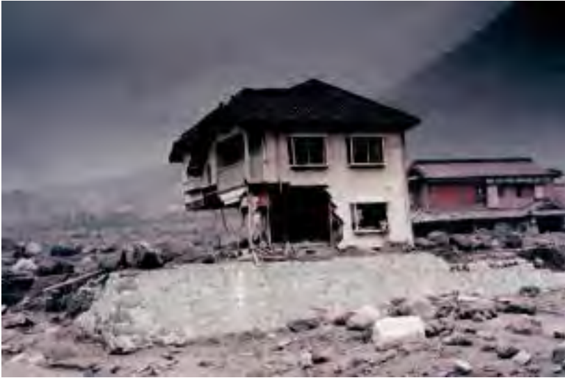
House damaged by a volcanic mud slide (lahar) in Japan.
