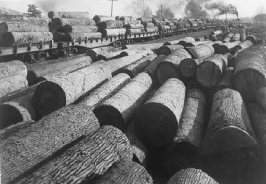
Plate 9.4 The railroad provided mass movement, versatility, and speed to the industrial logging process and was particularly important in the largely riverless areas of the South, as depicted in this photograph taken in Arkansas circa 1904. (Forest History Society, Durham, N.C.)
