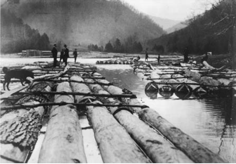
Plate 9.3 Industrial logging: rafting yellow poplar logs on the Big Sandy River, Ohio, circa 1920s. This was a small operation in a minor timber-producing area, but it illustrates the principle of fixing logs together, which on the larger rivers of the continent produced rafts of up to 5 acres in size, pushed and nudged along their journey by steam-powered riverboats. (Forest History Society, Durham, N.C.)
