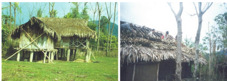
Photo 2 Chakma house made of bamboo, wood and roofing with Zalacca Secunda leaves
