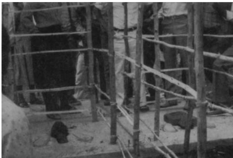
FIGURE 27 Latrines under construction.
