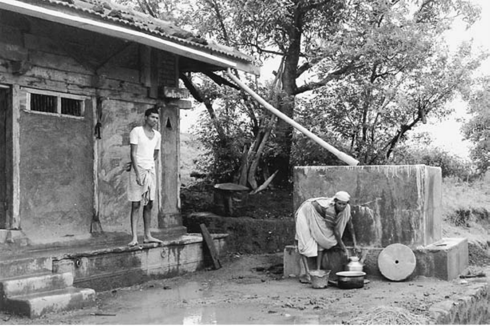
FIGURE 4 Roof water harvesting Manhere Village, Akole Taluka , Ahmednagar District, Maharashtra State, India.
