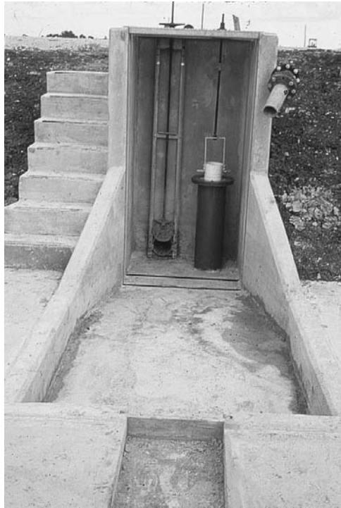
Figure 7. A concrete kettle with a catch basin in front. Note the stairway to the left, the valve that can be opened to completely drain the pond, and a moveable (up and down in this case) standpipe to control the water level when the pond is in use or being drained. The pipe on the right side of the kettle is an inflow line. The screens have been removed in this photograph.
