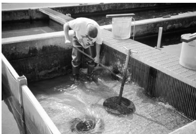
Figure 5. Some of the solids swept from a raceway's fish-rearing area can settle in quiescent zones, but the captured solids must be manually removed. Shown here is a quiescent zone being cleaned at the Pennsylvania Fish and Boat Commission's Big Spring Fish Culture Station (Newville, PA), where it takes about one day for a single person to clean all 80 of the hatchery's quiescent zones.
