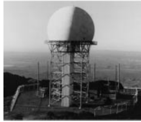
Fig. 21. The ARSR-4 is a long-range, three-dimensional, solid-state surveillance system. It was specifically designed as a joint-use radar for the FAA, the US Air Force, and the US Navy. The ARSR-4 detects all aircraft out to 463 km through all weather and clutter conditions as well as man-made interference. Photo courtesy of Northrop Grumman Corporation.
