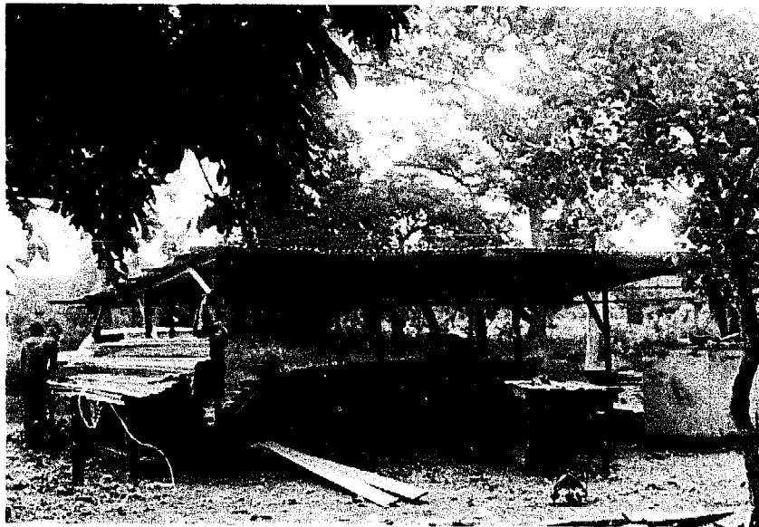
Fig.19 Chantier artisanal Fig.19 Artisanal boatyard
