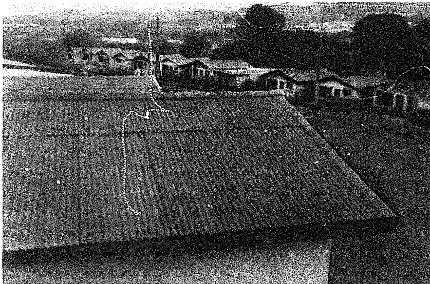
Fig. 5.15 Asbestos cement roof.
