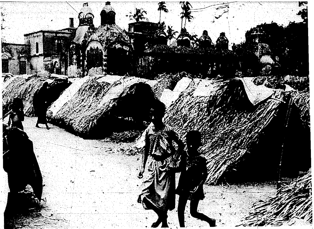
At right: the Amdanga refugee camp was set up in a temple courtyard in India, during the Bangladesh disaster. 30,000 refugees stayed here in simple A-frames with thatch covering.
