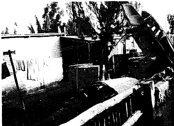
FIGURE XII. EXTENSIONS AND ADDITIONS ARE MADE TO THE HOUSES
