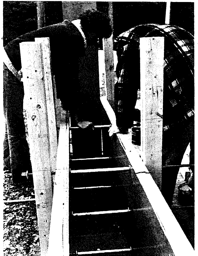
Spacers and washers must be placed inside of the forms.
