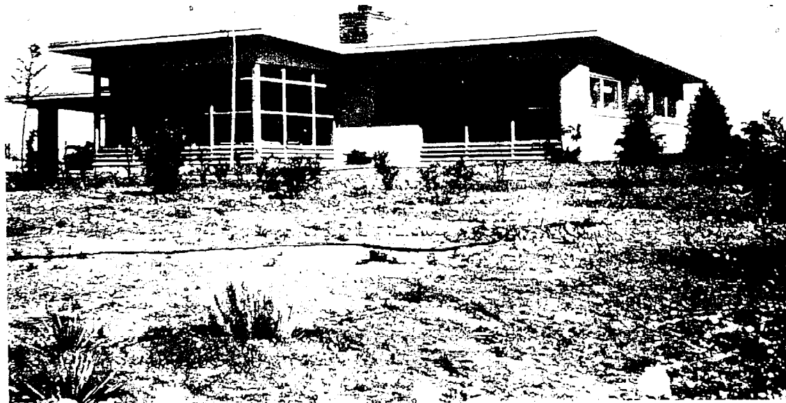
EXTERIOR SURFACING on Miller house consists of dagga-cement plaster, brush-finished with water-proofing and finished with a cement base paint. Local failures in this finish led to tests of new formulae.
