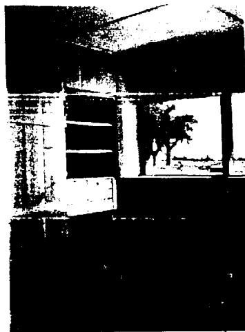
SINCE INTERIOR WALLS are exclusively formed by story-high cases of various sorts, the house has an unusual amount of storage space. Interior surfaces of earth walls are dagga plaster, waterproofed and then brushed with one coat of oil paint.
