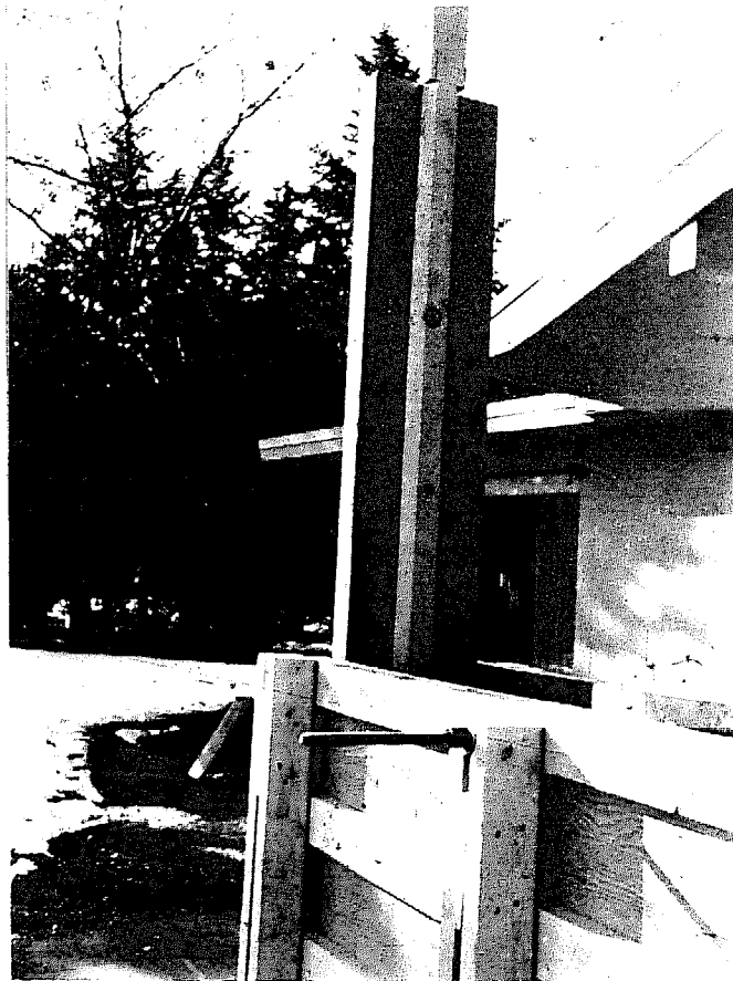
Beveled 2"x4"x10' nailed on center of inside of endgate; 12" wide for 12" wall.
