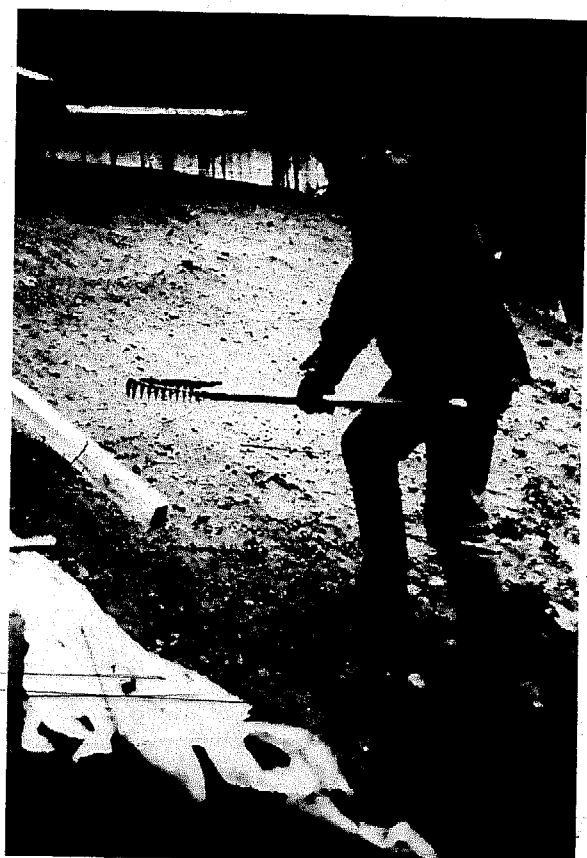
Incorrect procedure for raking first layer of earth smooth is demonstrated here. Tines of rake should not be used, but backside, so as not to risk tearing polyethylene.
