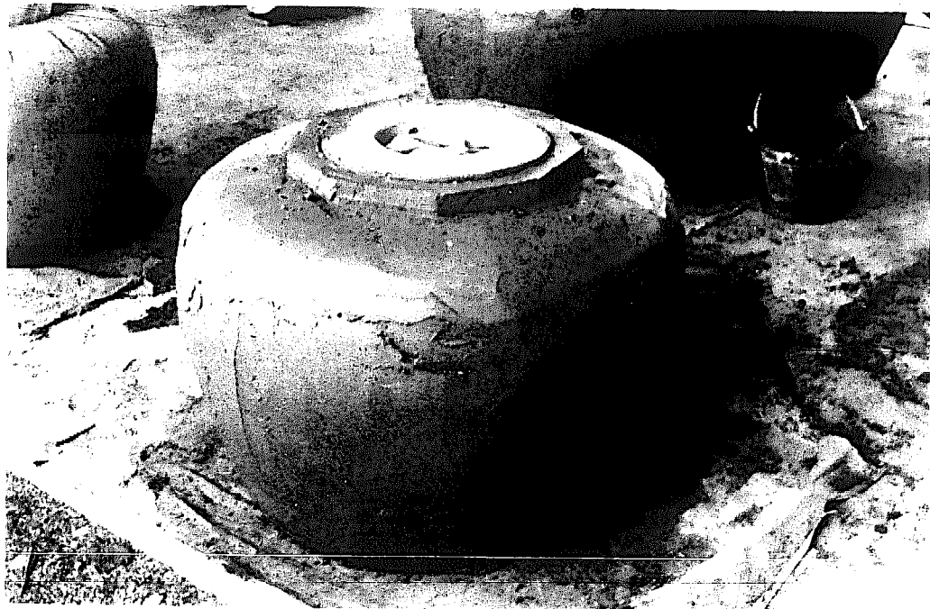
Figure K8: The first layer of cement mortar is applied from the bottom to the top with a thickness of about 0.5 cm.
