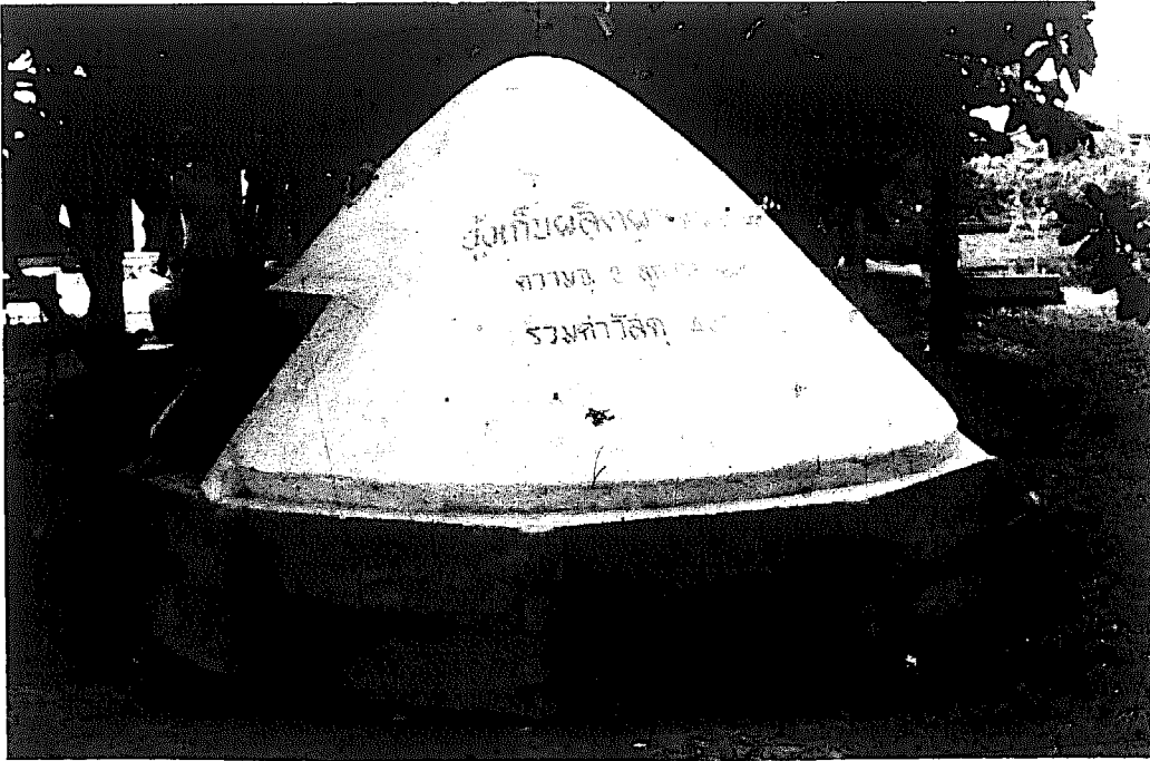
Figure G1: Completed cement mortar bin
