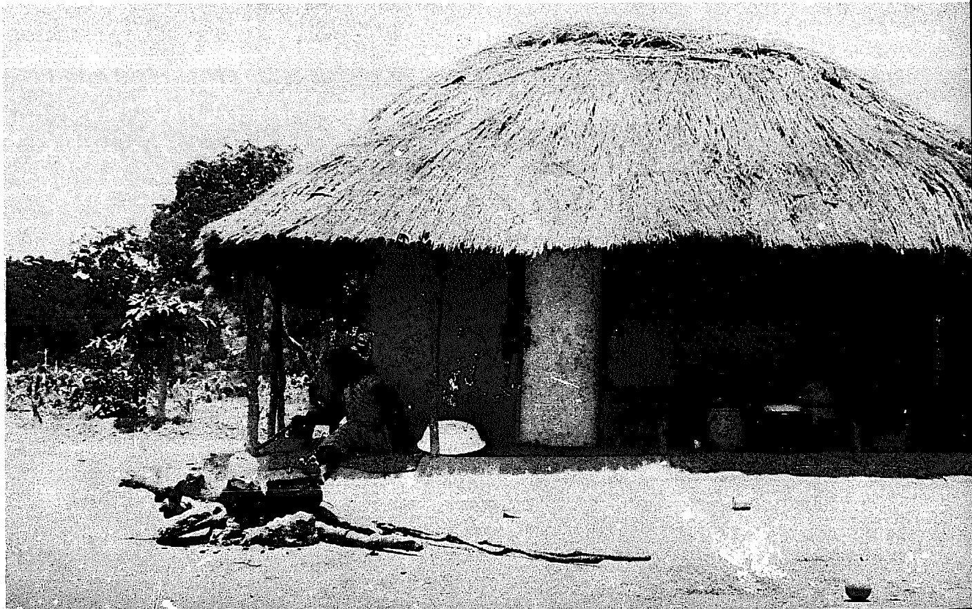
One of the more substantial pole and dagga houses of Shillinga Kaseba which was replaced with a stabilized earth brick structure.
