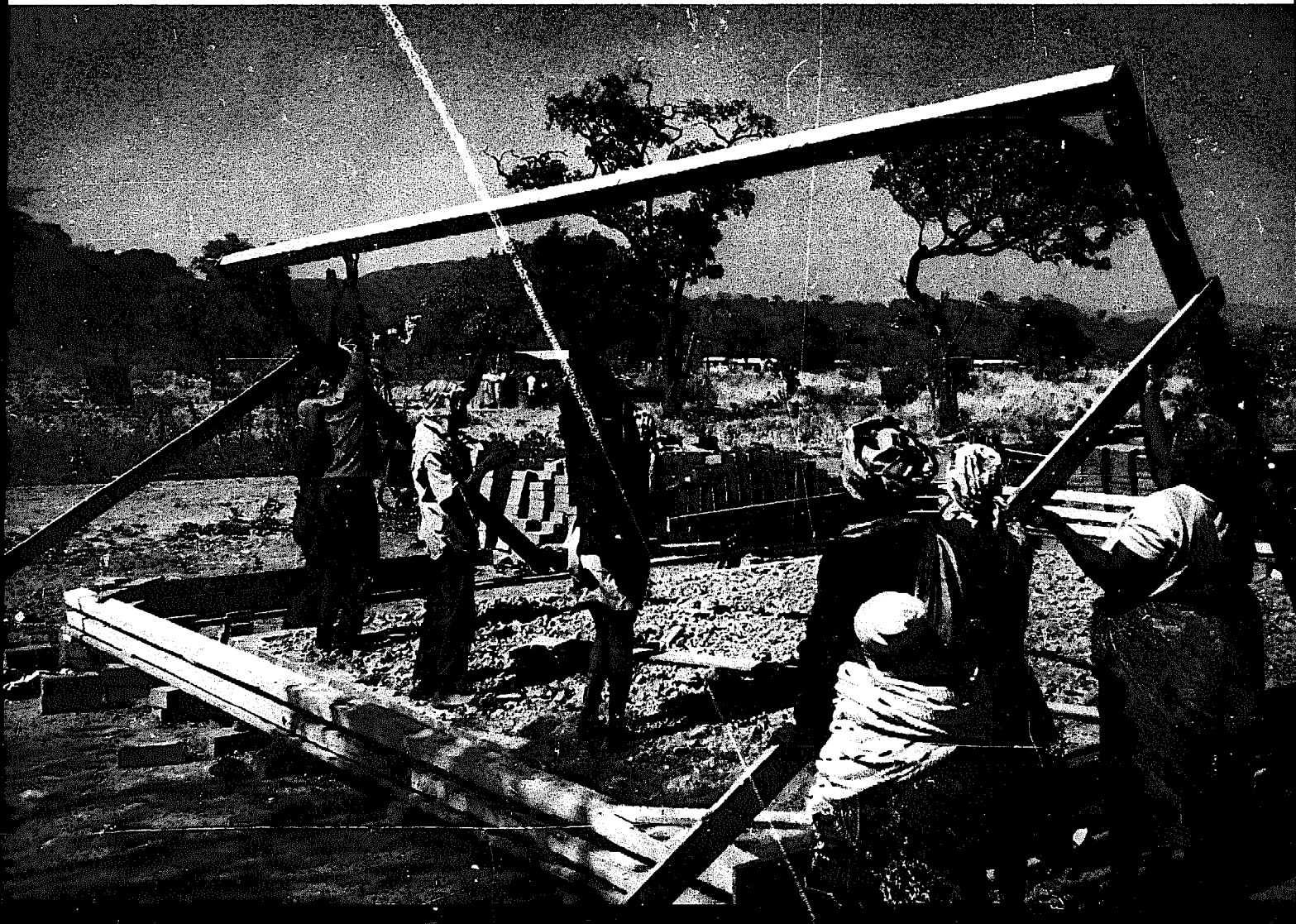
Raising the frame that will support the roof so that work can progress through the rainy season. The frame also aided in keeping the walls square and plumb.
