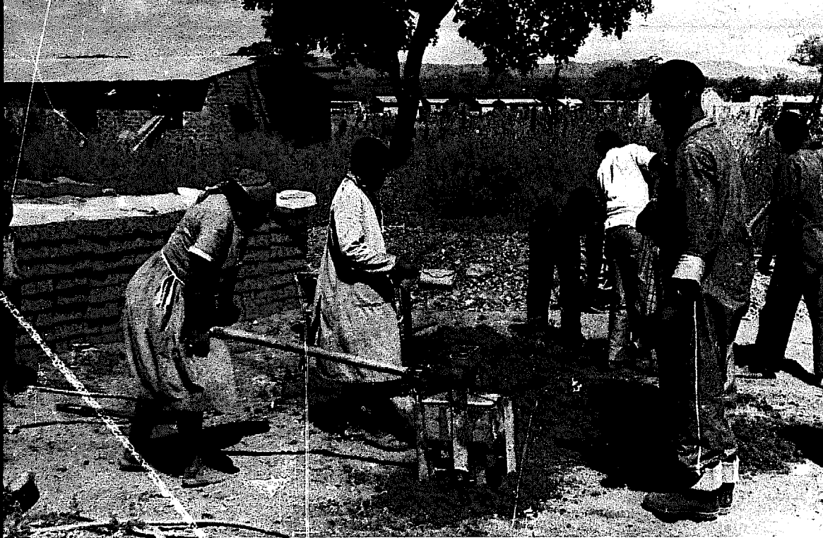
Pressing the earth and cement mixture in the Cinva-Ram which produced the bricks.
