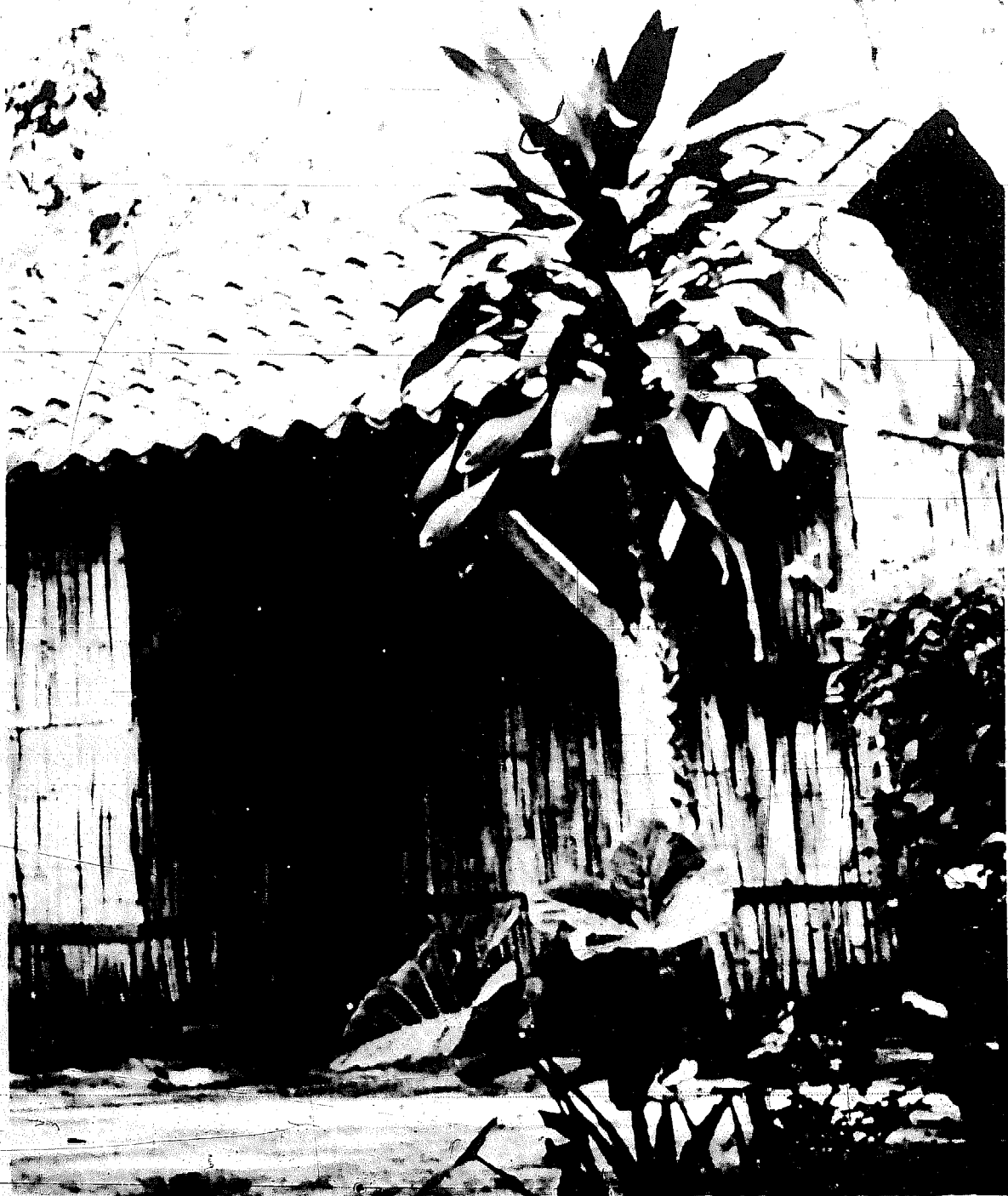
Figure 20.--Tile covers the roof of this bamboo house in Guatemala. The "boards" of the wall are made from culms of Bambusa vulgaris .
