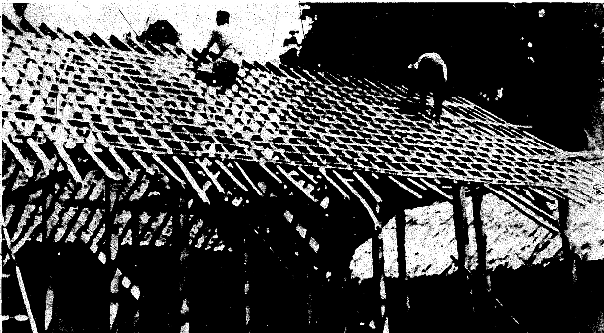
Figure 4.-- Framework of this house under construction in Java is hardwood; but rafters, sheathing, scaffolding, and even the ladder are bamboo. Walls and partitions may be covered with bamboo matting, probably made from species of Gigantochloa , commonly used in Java for this purpose. (Photo by Dorsett.)
