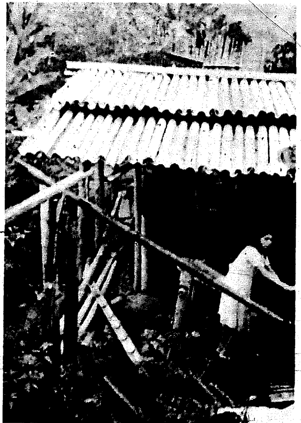
Figure 19.--Roof tiles of this laundry in Colombia, as well as the troughs of its water system, are halved culms of Guadua angustifolia , the common native bamboo of Colombia and Ecuador.
