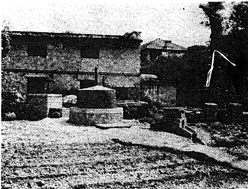
The same plant in operation
