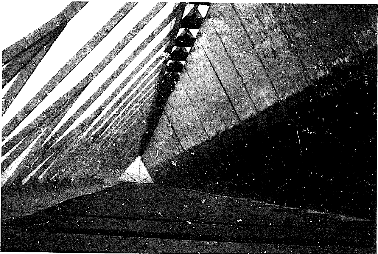
Figure 4. View of Insulator-Reflector in Raised Position
