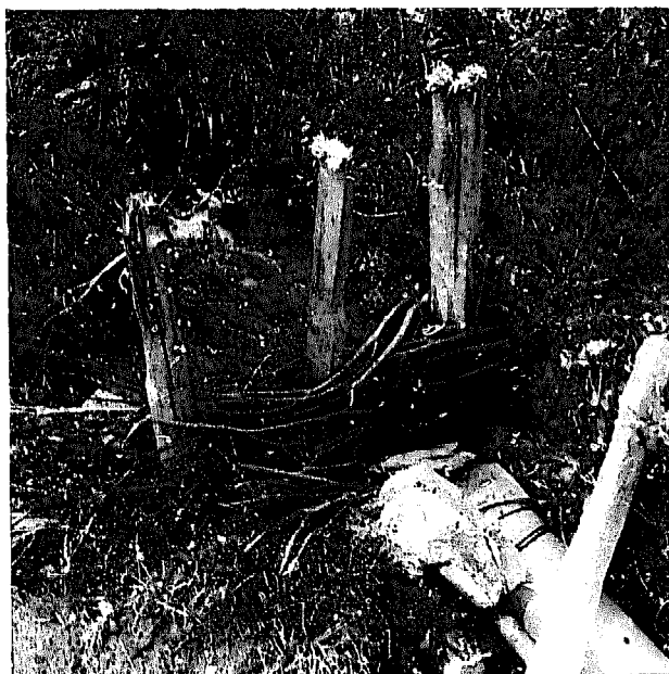
Fig. 3: Simple water intake in a marshland below the spring (no floods, no debris load).
