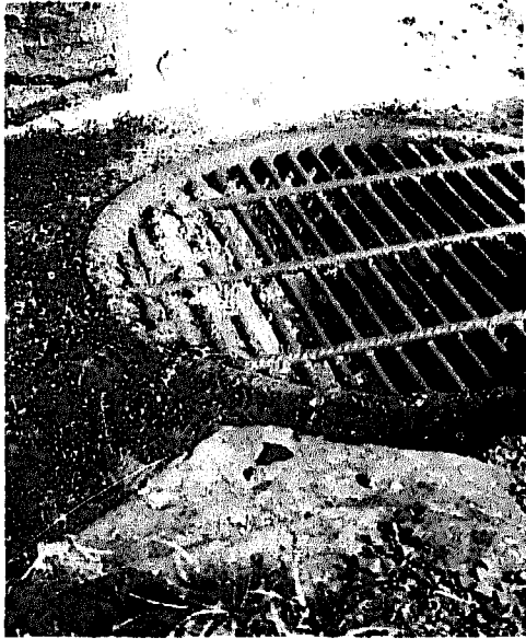
Fig. 13: A simple intake consisting of a trash rack made of concrete reinforcing steel, placed on a concrete pipe (inside dia. 100 cm) which is dug into the bed of the stream.
