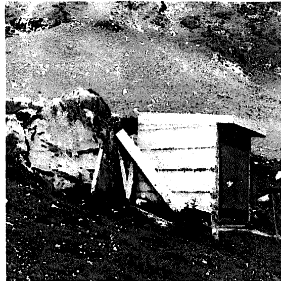
Fig. 22: The machine house stands in an avalanche prone area, protected by a rock.
