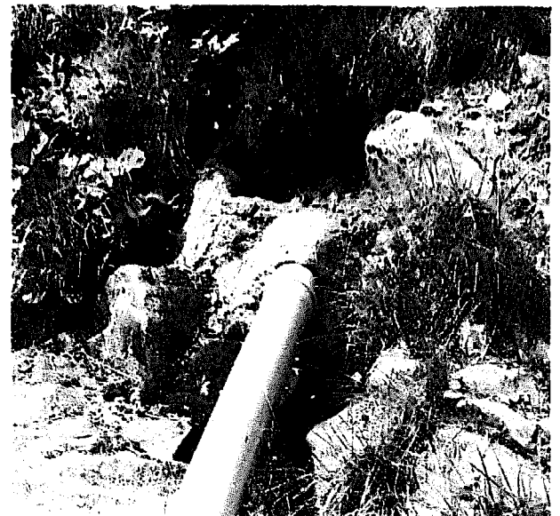
Fig. 8: Spring kerb: Immediately after emerging, the water is collected in a concrete basin and is led into a PVC-pipe (inner diameter 100 mm).
