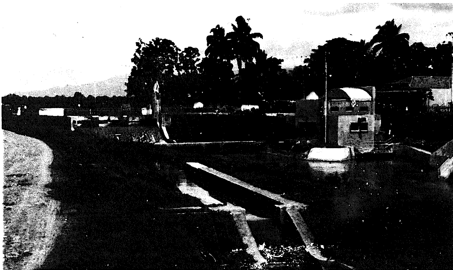
WONODADI, INDONESIA Low-head, 210 kW installation at a drop on an irrigation canal.
