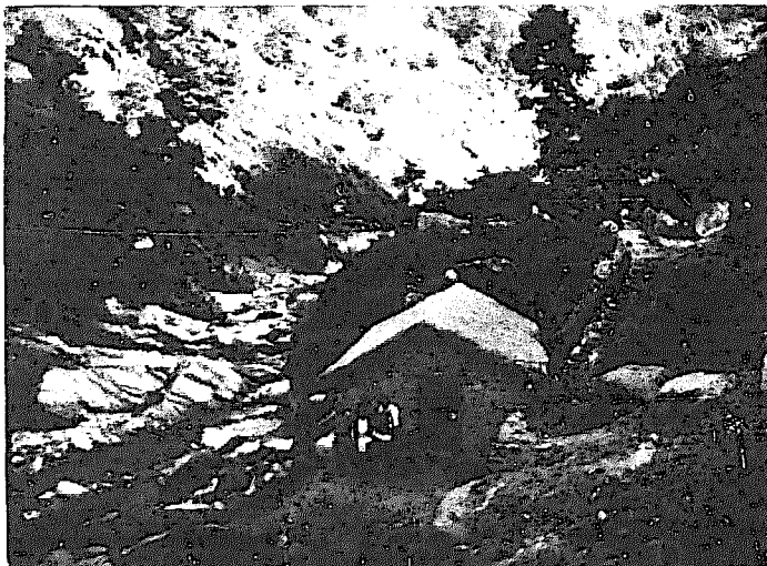
A new, small mill house with a MPPU in the hills. The low head requirements enables the installations at traditional mill sites.
