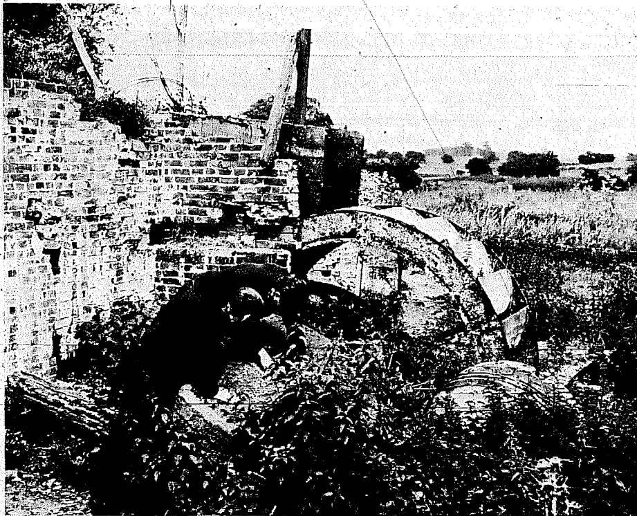
Fig 1.33 Overshot waterswheel in the ruined mill close to Churchover, near Rugby, Warwickshire. Note the remains of the wooden launder and 'shut' for bringing water onto the top of the wheel
