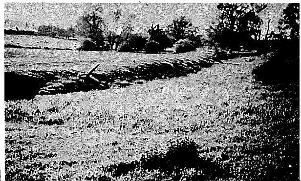
Fig 2.9 The artificial leat, made to serve Maidford Mill, on a tributary of the River Tove in Northamptonshire. The pentrough onto the overshot waterwheel is off the left of the picture. The natural course of the Maidford Brook is shown by the line of low hedges just in front of the field with sheep in the left background
