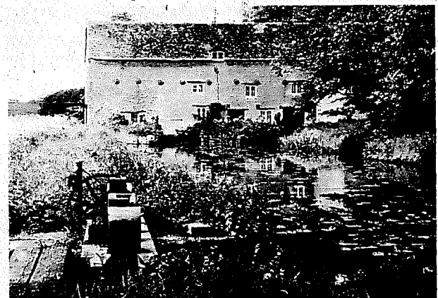
Fig 1.27 Wadenhoe Mill, near Oundle, Northamptonshire. The mill is situated on an artificial cut or leat and the main stream of the River Nene is navigable at this point. In the right foreground is the sluice for diverting water into the by-pass channel
