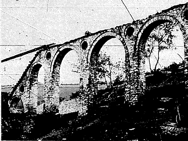
Fig 1.16 Some of the stone arches which used to support the series of connecting rods, the ends of each carried on wheels, which transmitted power to a bell-crank lever above the pump shaft, a quarter of a mile up the valley
