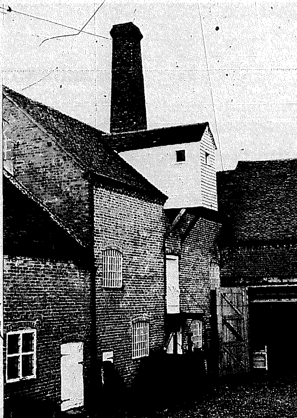
Fig 1.81 The white weather-boarded lucam, covering the external hoist, protruding from the roof at Sarehole Mill, Birmingham
