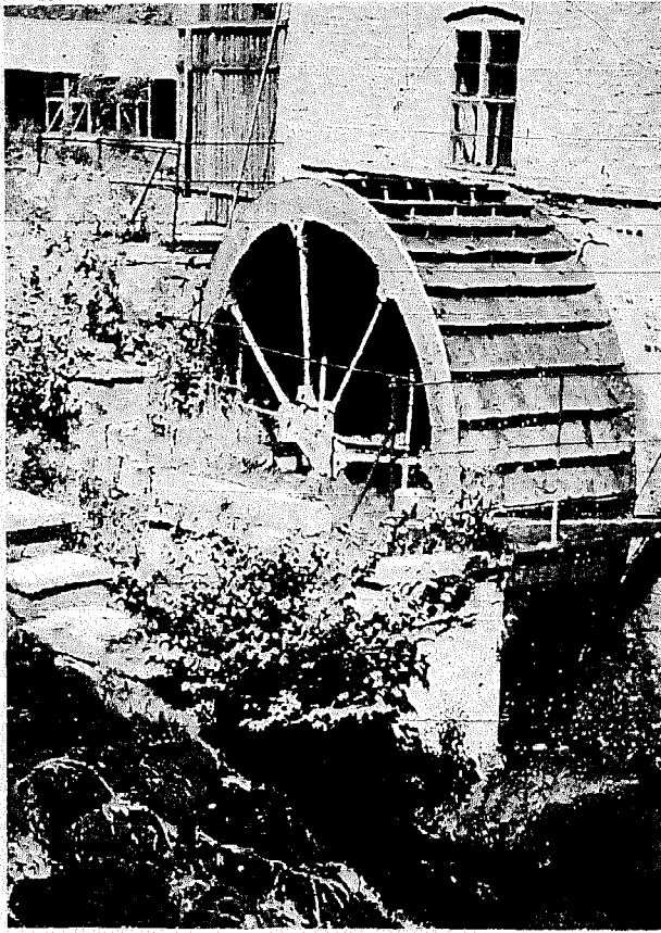
Fig 1.31 The breastshot wheel which used to drive the corn mill at the end of Arkell's Dönnington Brewery, near Stow-on-the-Wold, Gloucestershire
