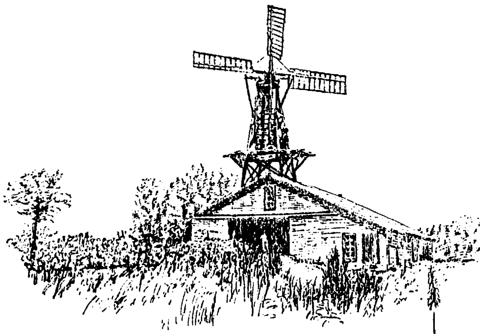
FIG. 54. The large Dutch mill built by Mr. August Prinz, Chalco, Nebraska. Diameter of wheel thirty-six feet; capacity two hundred to three hundred bushels of ground feed a day, according to the wind; efficiency between six and eight horse power. Runs an eight horse-power feed grinder. Cost $150. The designer prepared his own models, and had them cast in Omaha.
