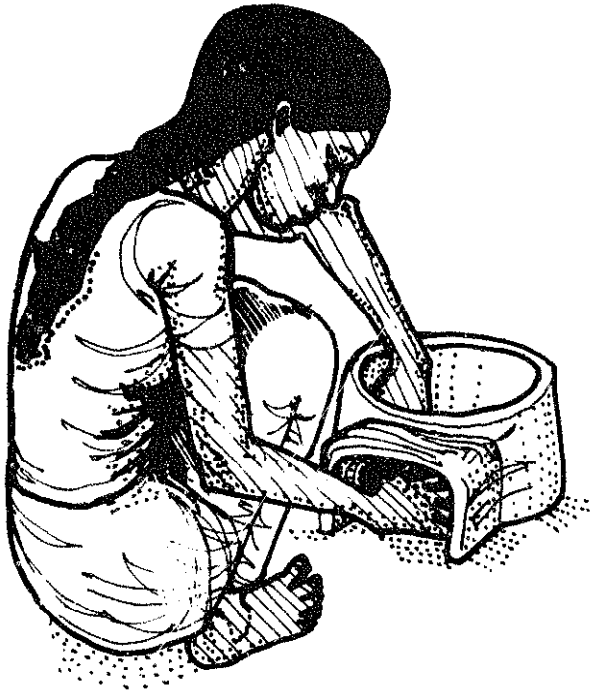
The door arch is coiled on to the firebox
