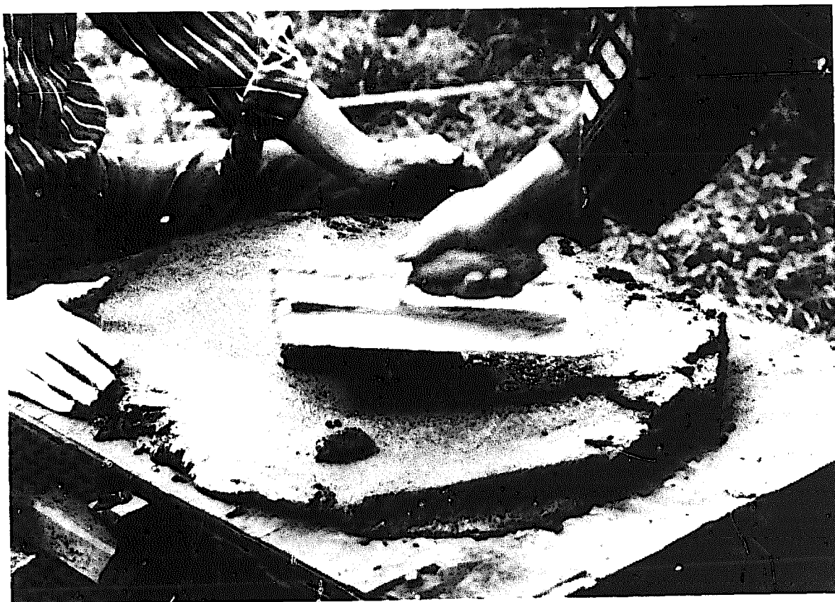
Building a Lorena stove: applying the first layer of lorena
