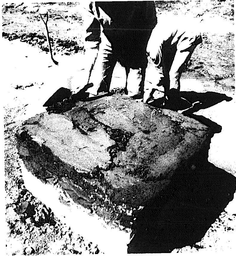
Applying the fourth layer of lorena
