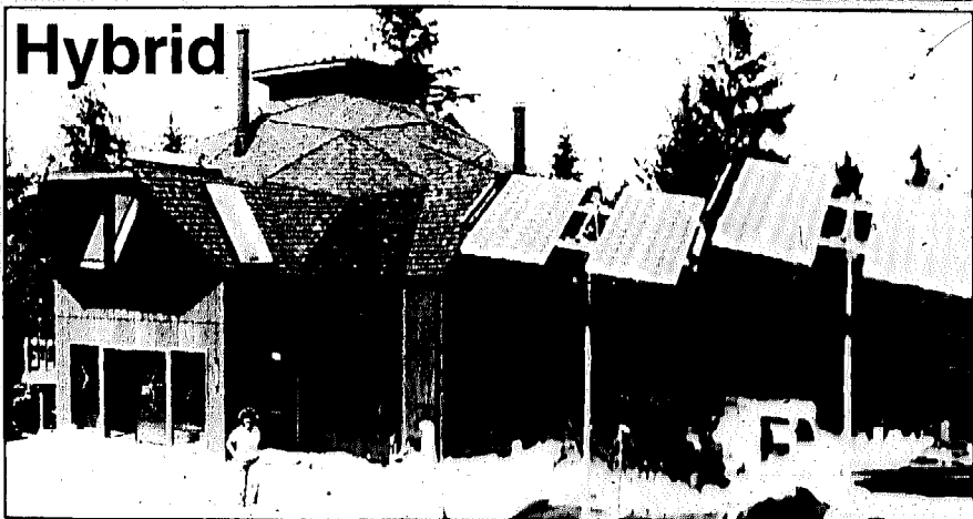
Eight ARCO panels follow the sun with the help of two Zomeworks passive trackers, providing enough power for up to seven sunless days for Walter and Eddy Ross.
