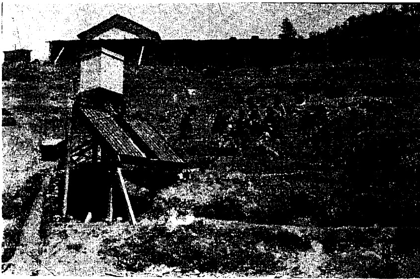
Solar water heater installation in Chialsa, in the remote hills.
