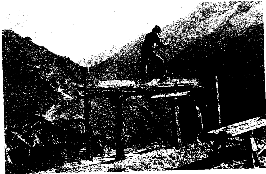
Cutting of wood with a log saw is a welcome improvement over traditional methods still using axes.
