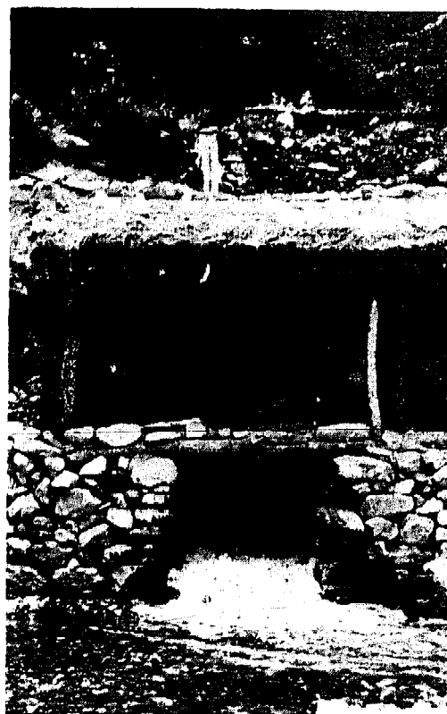
Front view of a typical traditional mill house.
