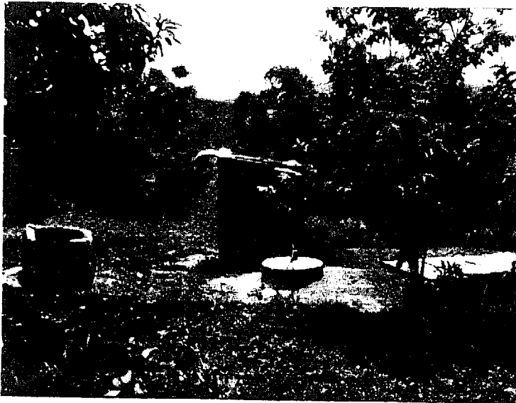
A completed underground digester, here in combination with a latrine. (Ref. 36)
