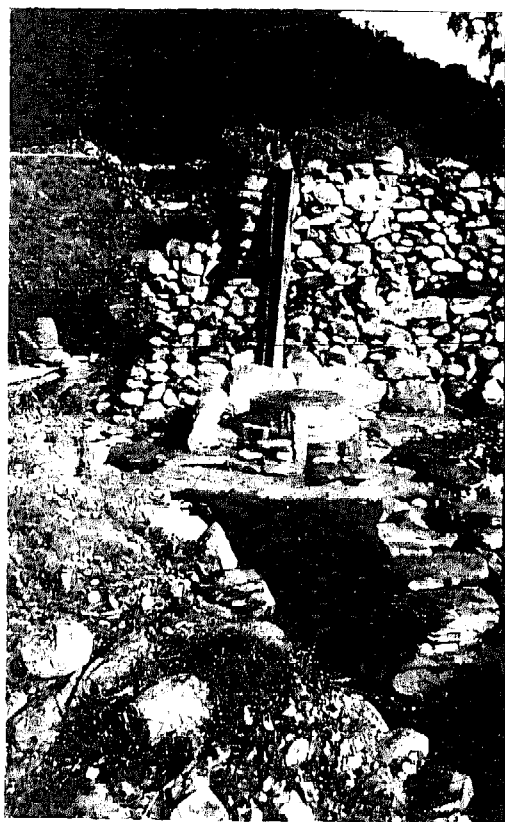
A new construction of a traditional horizontal water mill in the hills.
