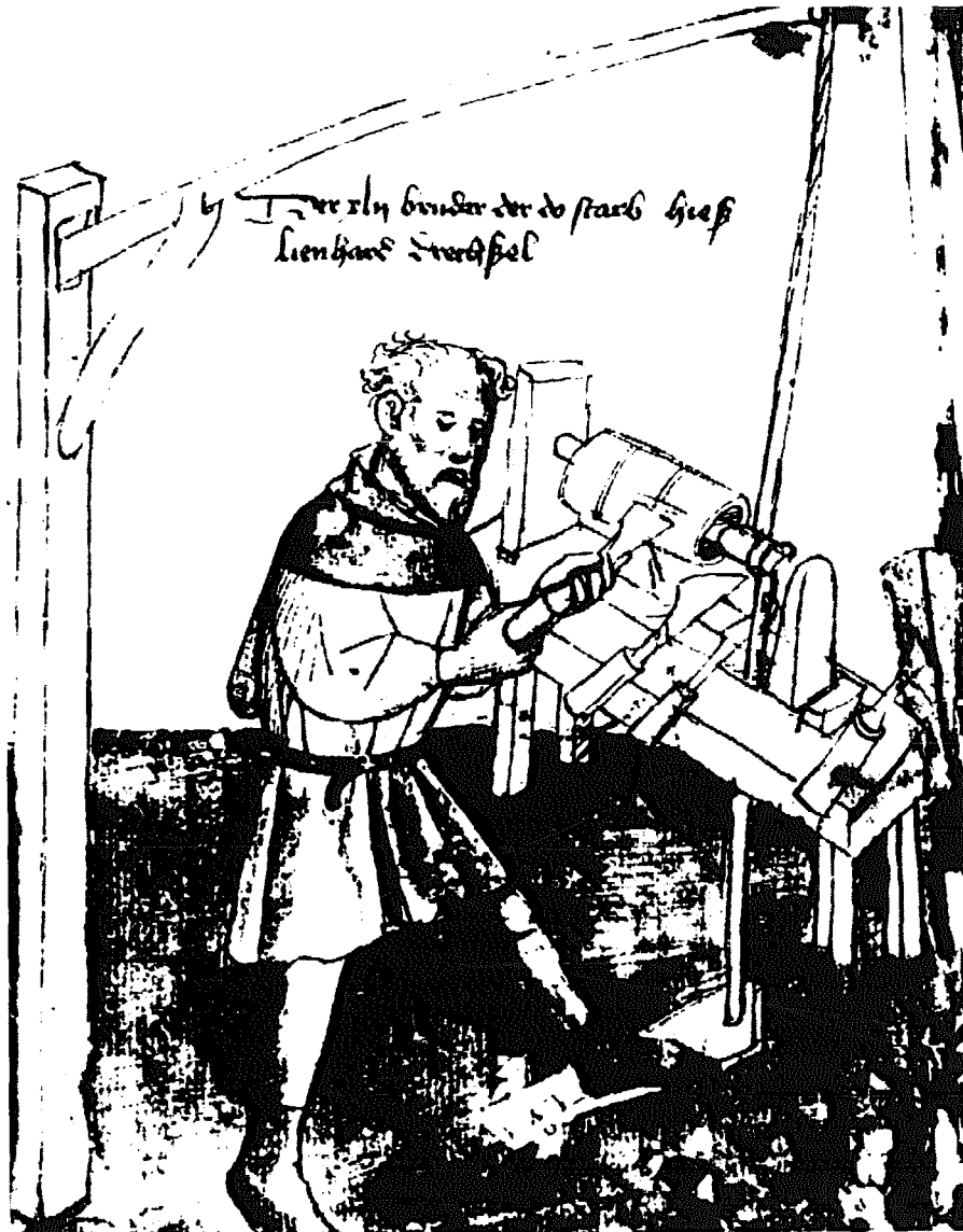
Figure 1-18 Foot-powered lathe (Courtesy of Friedrich Klemm)
